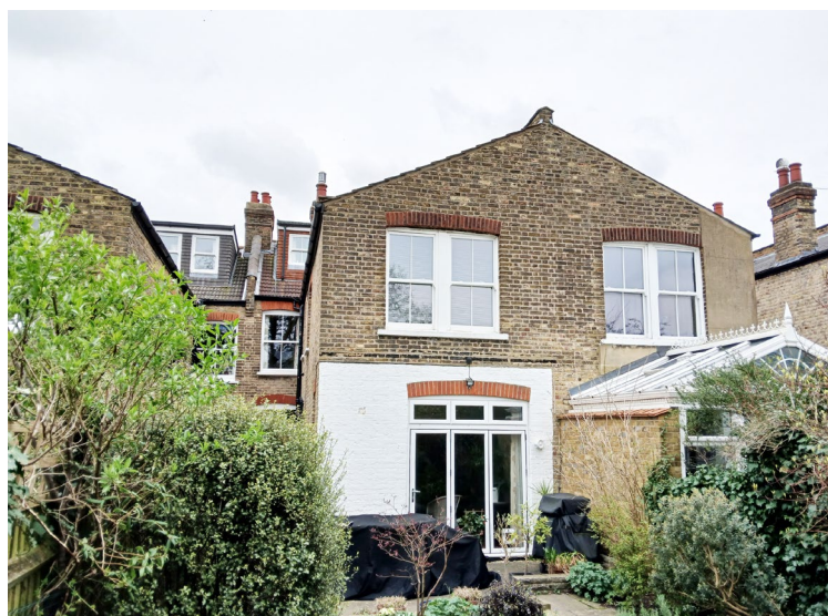
Rear view with neighbouring rear extension
