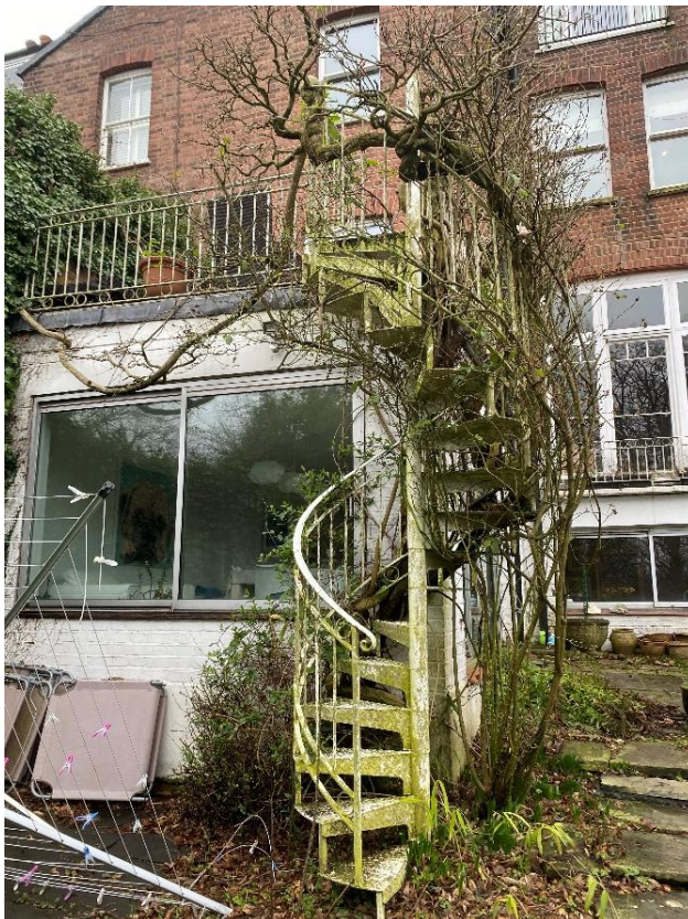
Photo 1: 60 Muswell Hill Road Existing Rear Kitchen Extension with spiral staircase.
