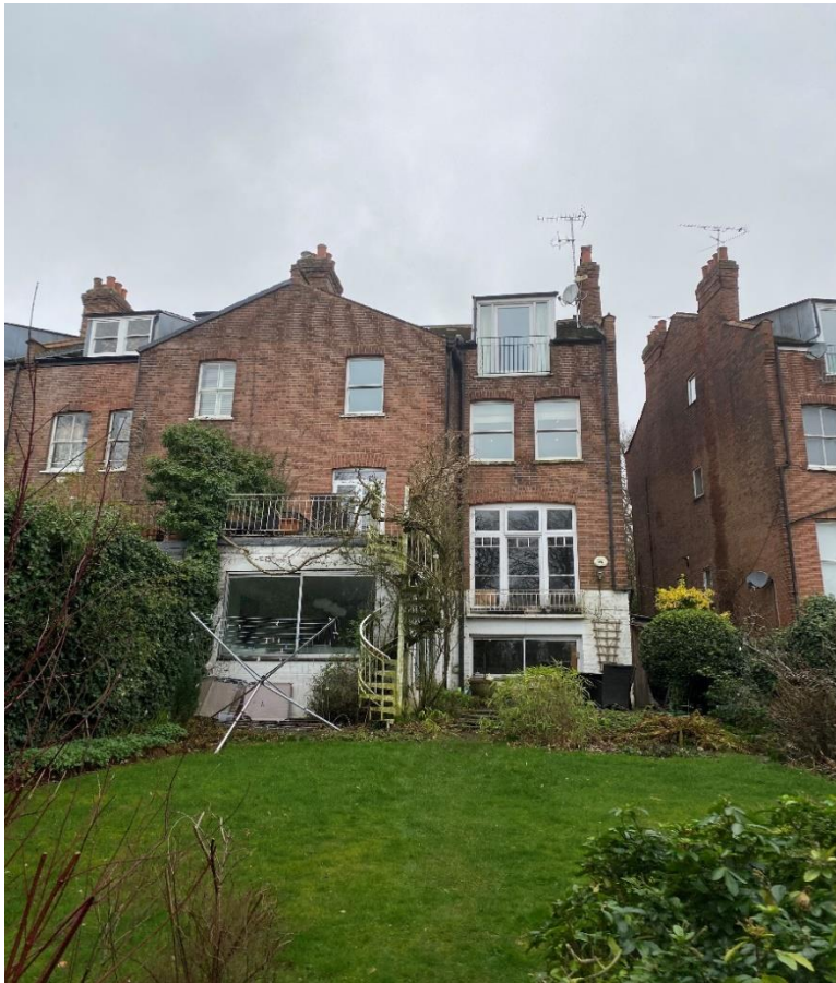
Photo 2: 60 Muswell Hill Road. Existing rear flat roof rendered kitchen extension with roof terrace.
