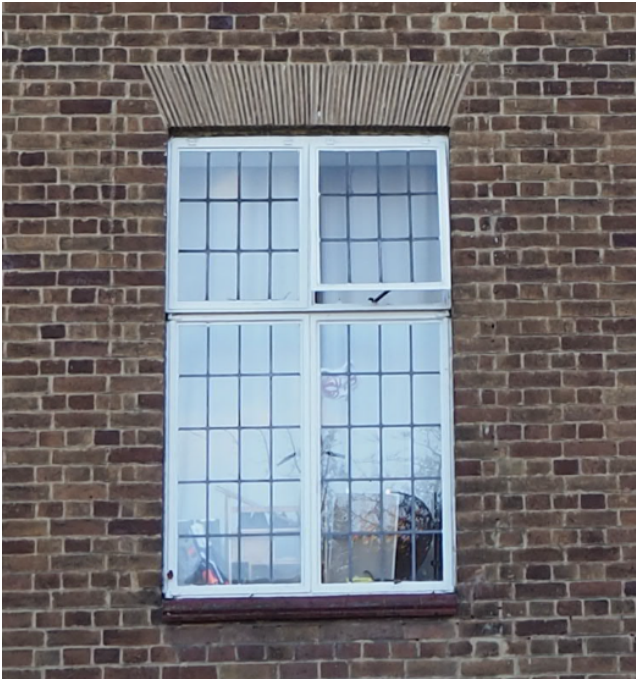
EXISTING WINDOW ELEVATION - EXTERNAL (single-glazed)
