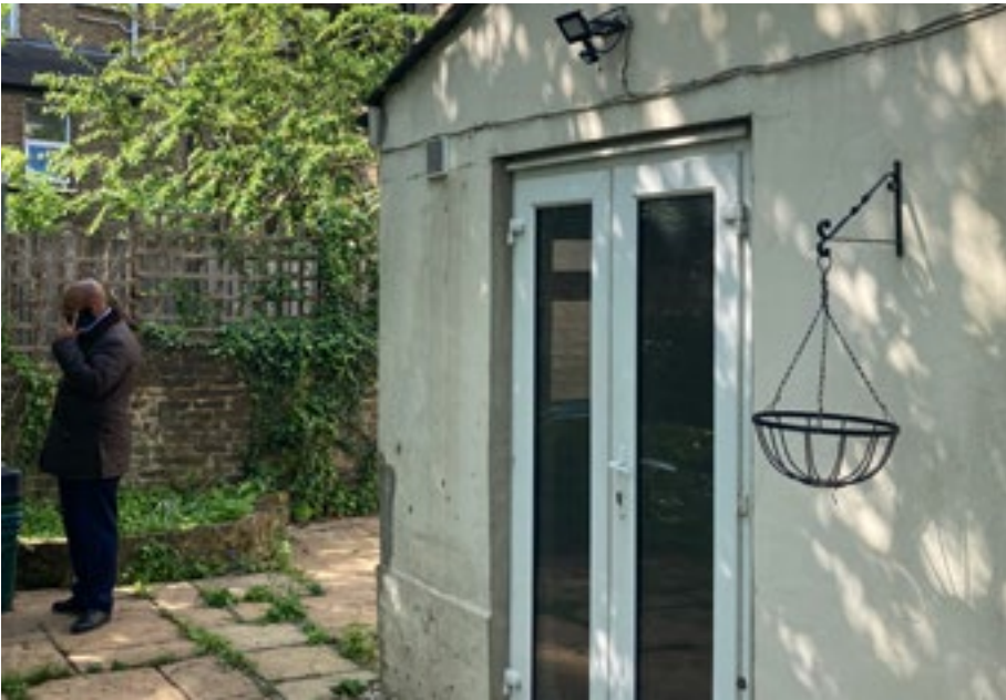
3. East facing facades
