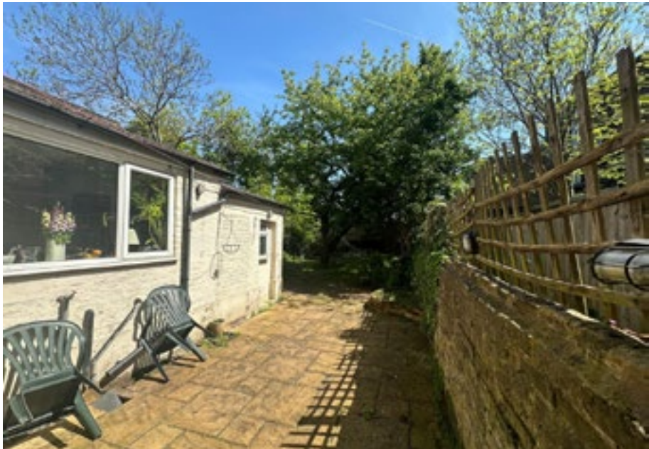
1. Existing southern facade of primary extension
