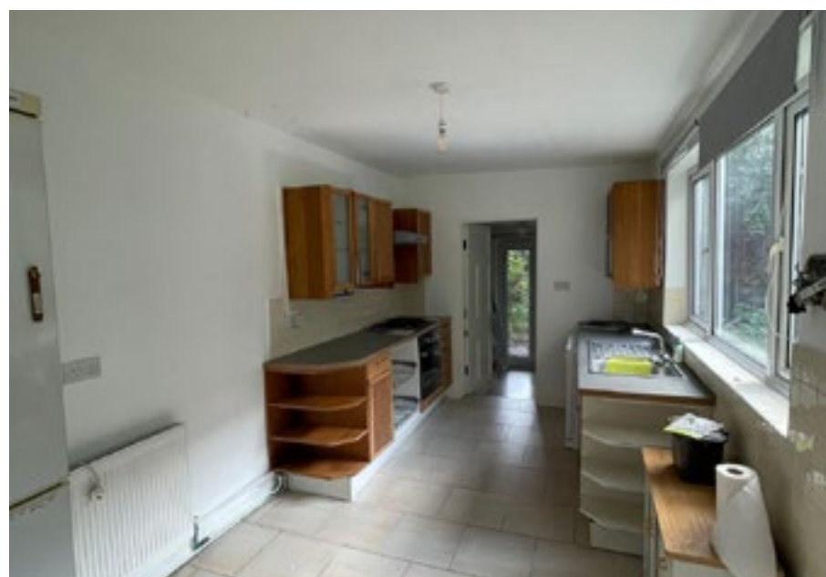
4. Existing outdated Kitchen extension
