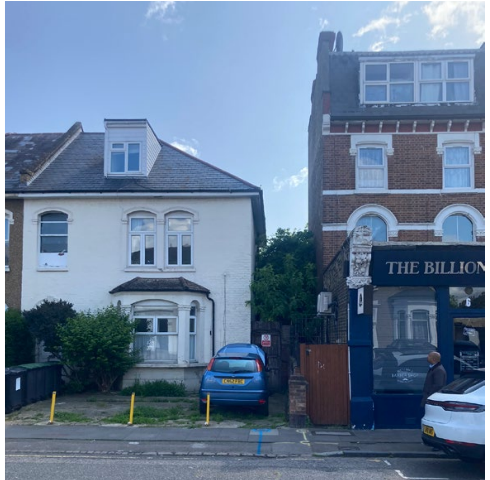
Photo of existing building on 8 Alexandra Road
