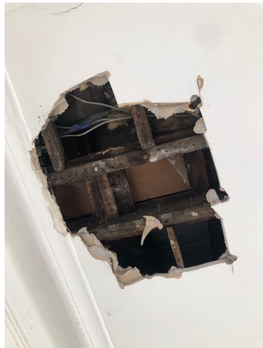
Figure 1: Modern plasterboard finish to the rear room ceiling.
