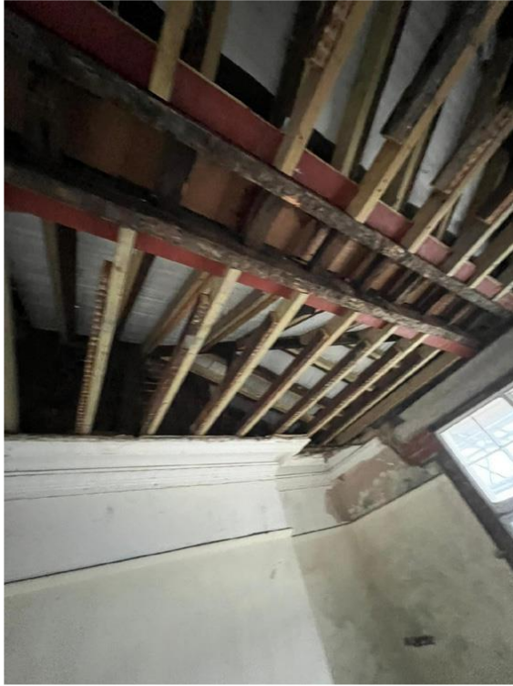
Above Left: Photo of new steelwork above rear room with chimney breast shown in foreground
