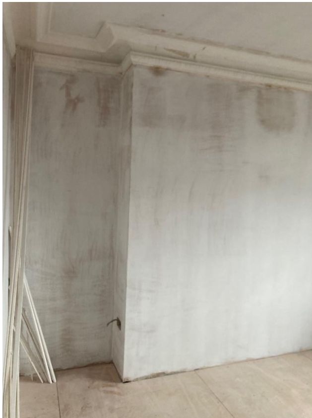
Above: Photo of chimney breast wall with ceiling and cornice reinstated.
