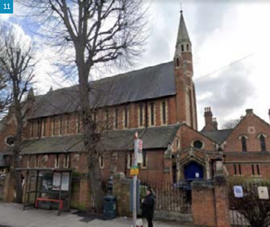
St Mary's, Lansdowne Road (March 2022 streetview)
