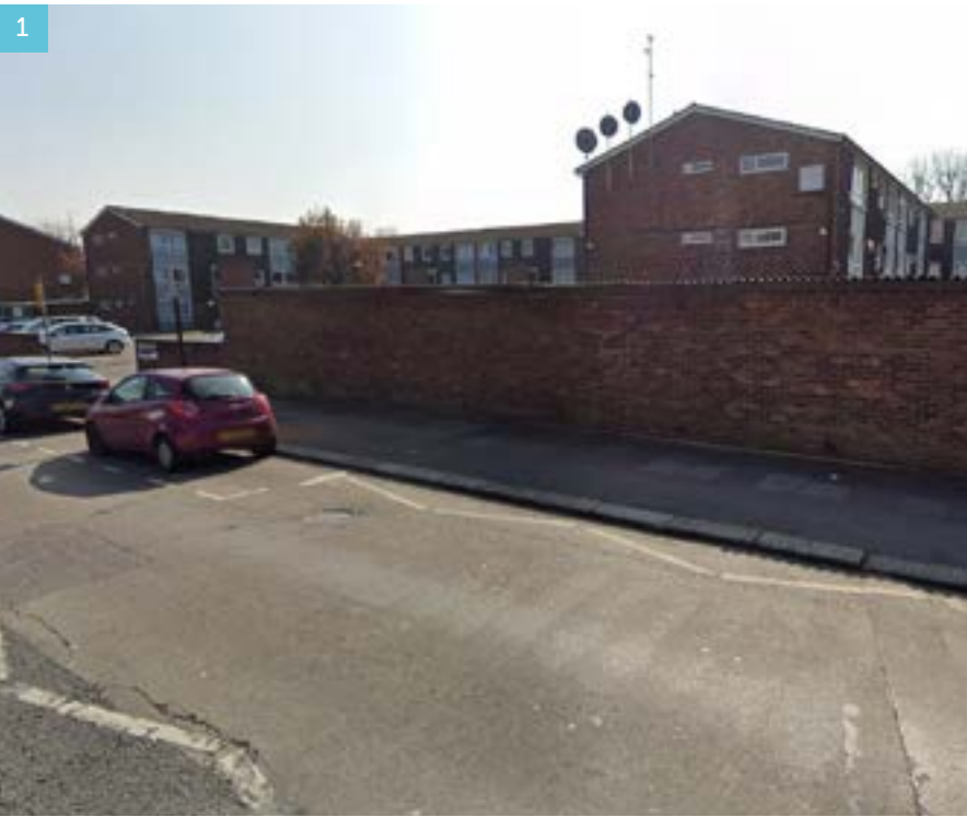
View looking towards the existing garages wall from Lansdowne road
