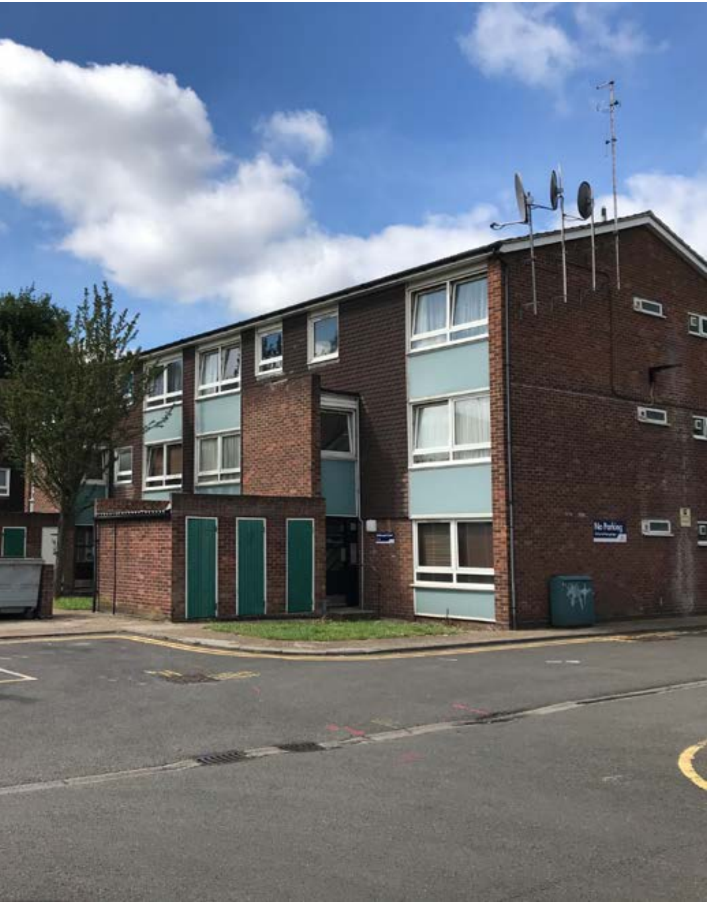
View of Baldewyne Court Courtyard looking South.
