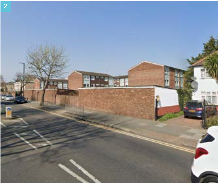
View looking West along Lansdowne Road
