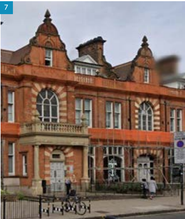
The Tampery Tottenham, 639 High Road N17 8AA - diagonally opposite the end of Lansdowne Road
