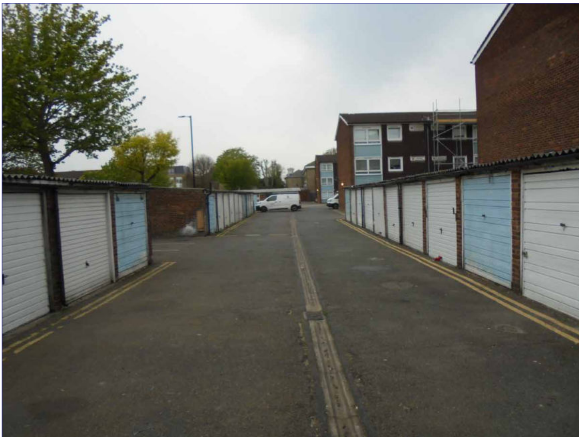
Plate 8: West facing view of garages on the south side of Arundel Court
