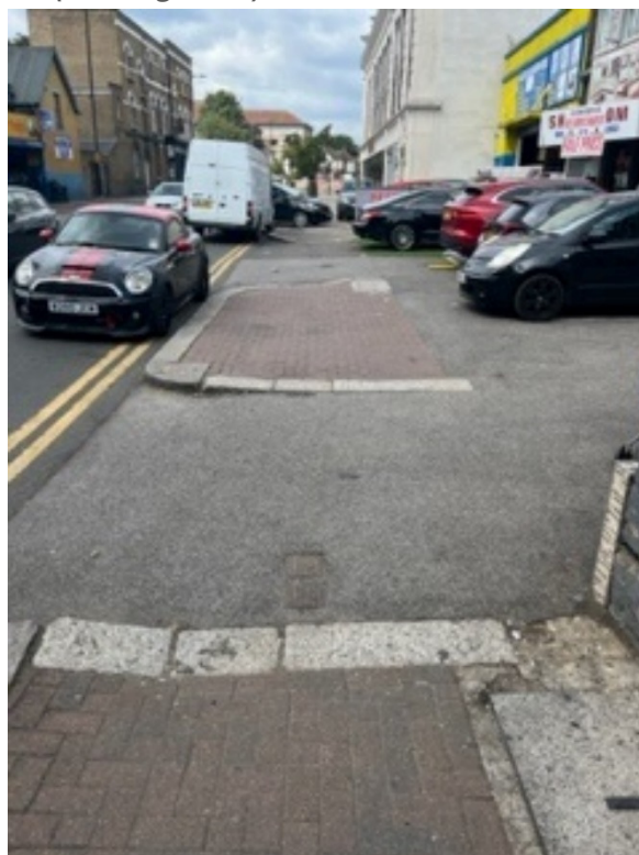
Photograph 4.1: Vehicular accesses and parking along the northern side of Lansdowne Road (looking west)
