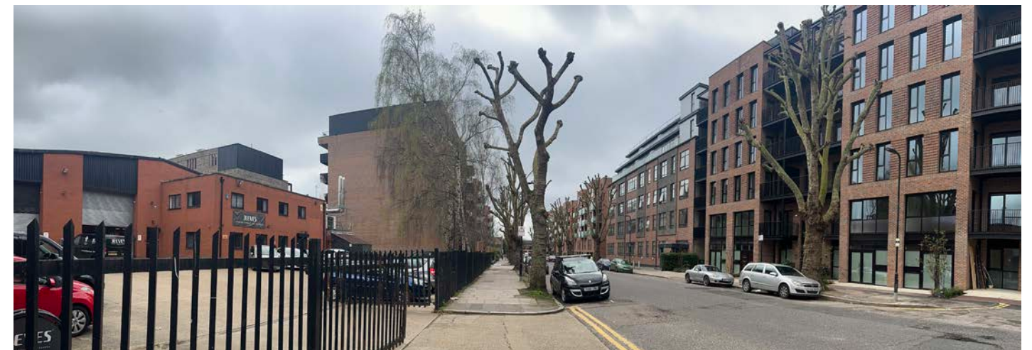
Figure 4.4 Panoramic view of the Site in context of adjacent new developments
