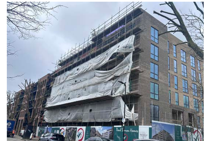
Figure 4.15 Plot opposite to the Site, currently under construction
