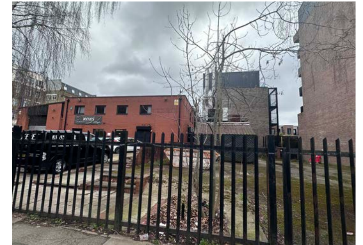
Figure 4.3 The poor street frontage along the existing frontage of the Site
