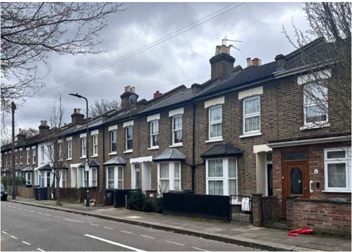
Figure 4.8 Homogeneous terraces along Collingwood Road, in Clyde Circus CA
