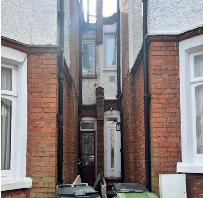
Front Facade - Side Access
