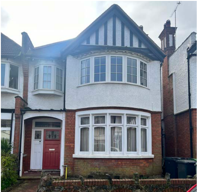
Front Street Facade
