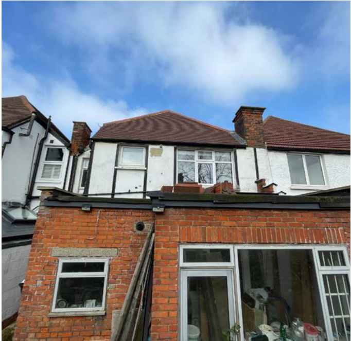
Existing Rear Facade
