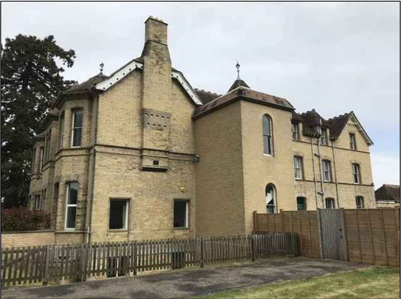
Photograph of Existing Elevation showing existing windows Brookthorpe Hall - Wynstones Lane, Gloucestershire
