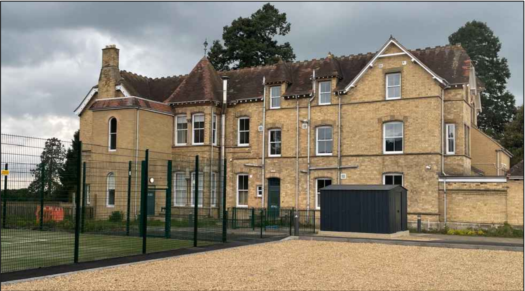
Photograph of As built Elevation showing new pvc-u sash windows Brookthorpe Hall - Wynstones Lane, Gloucestershire
