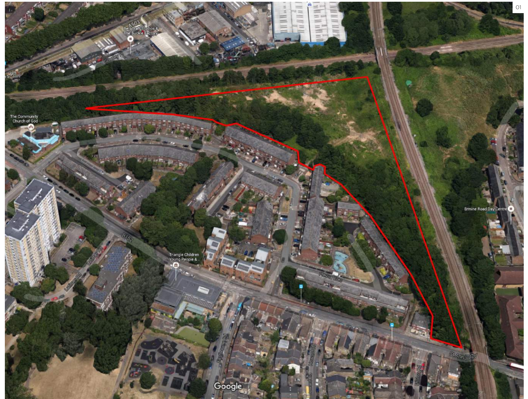
01 Site prior to development
