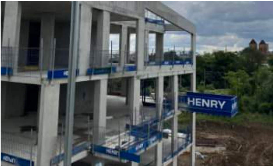
VIEW OF COMPLETED TOP FLOOR CONCRETE FRAME OF BLOCK C
