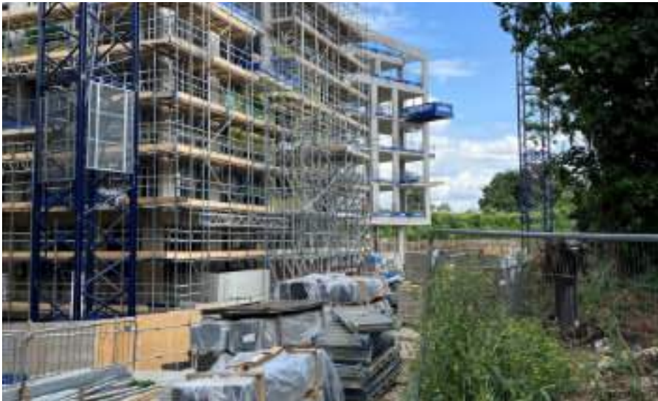
VIEW FROM SOUTH OF BLOCK A LOOKING TOWARDS BLOCK C
