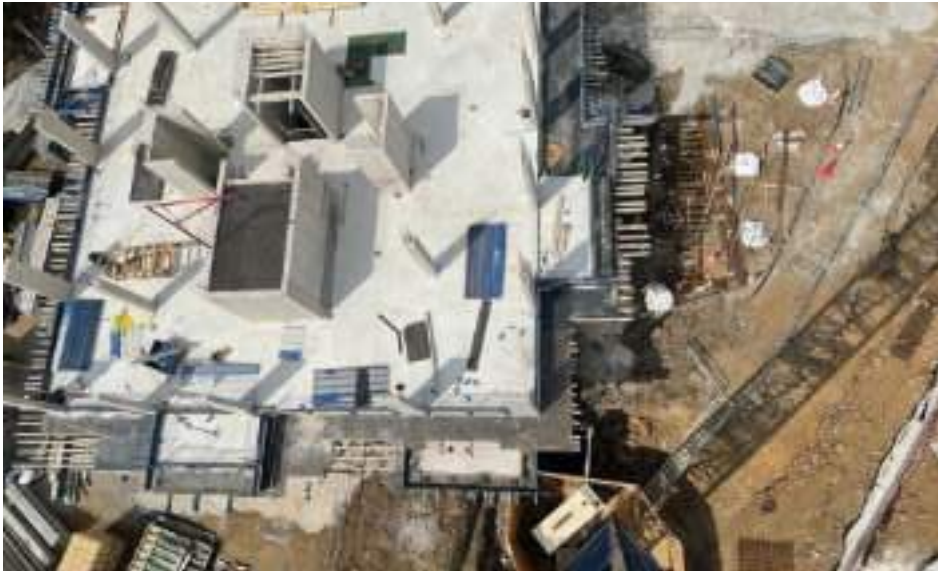
PARTIALLY COMPLETED FRAME SHOWING STAIR AND LIFT CORES
