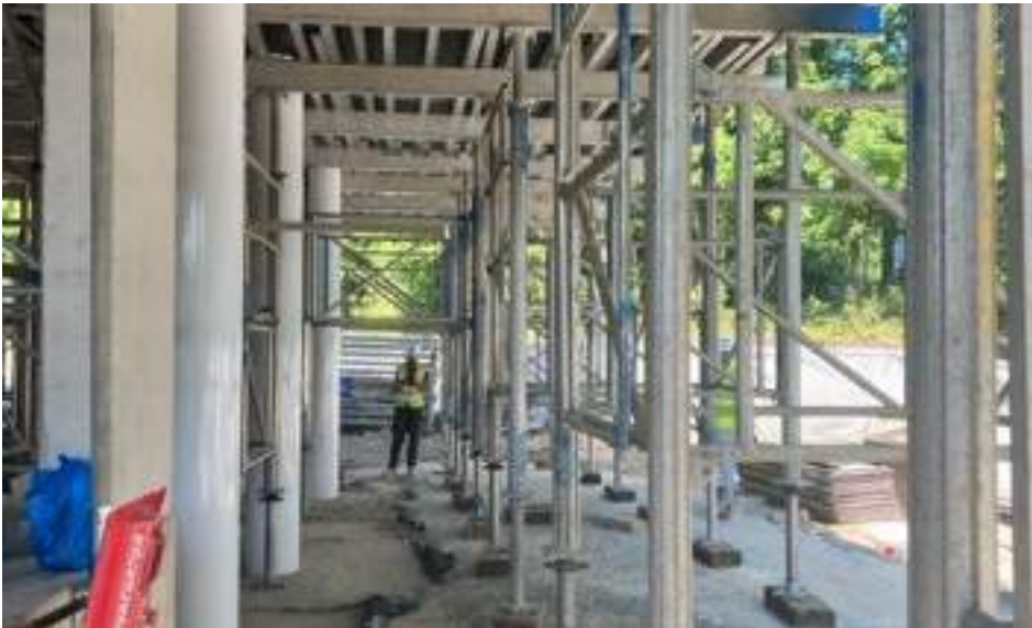
VIEW OF THE GROUND FLOOR ENTRANCE LOGGIA OF BLOCK A
