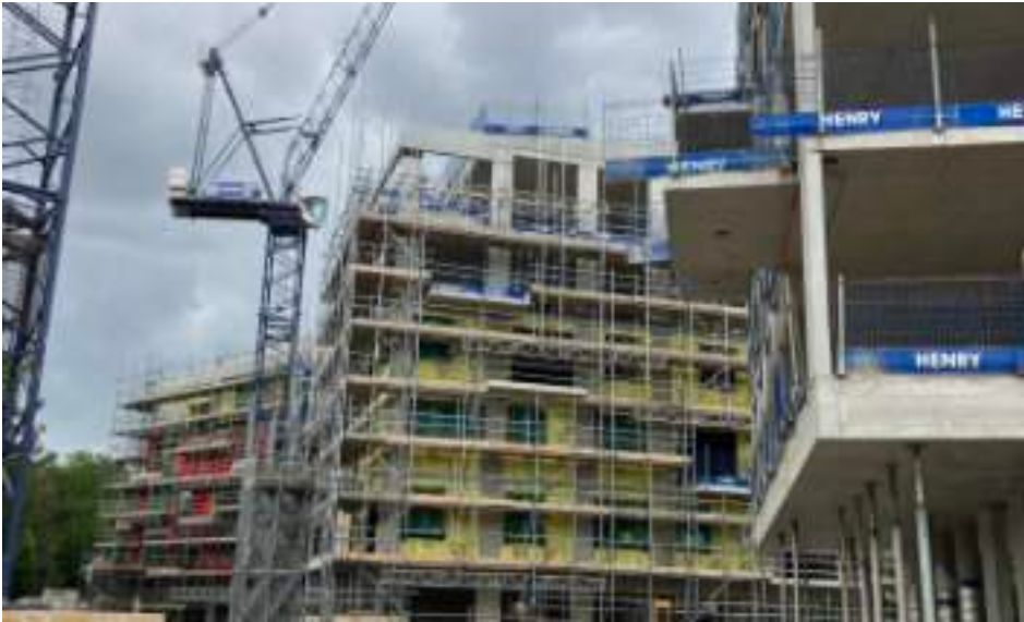
VIEW FROM GROUND LEVEL SHOWING BLOCK A (LEFT) B (CENTRE) AND C (RIGHT)
