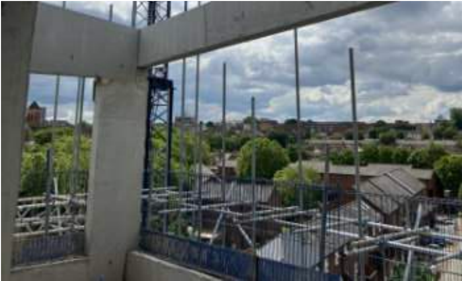
VIEW FROM INSET BALCONY ON THE TOP FLOOR SHOWING CONCRETE FRAMING
