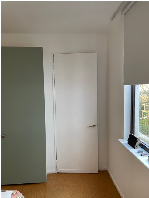
Non-original wardrobe (on left) projecting into bedroom
