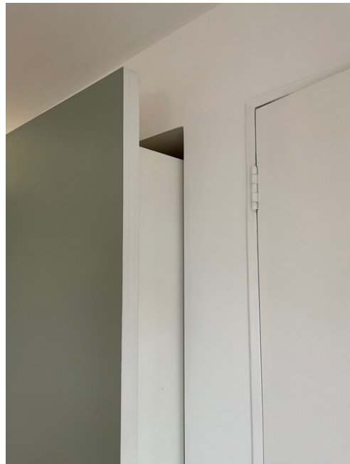
Detail of non-original wardrobe projecting beyond original cupboard line
