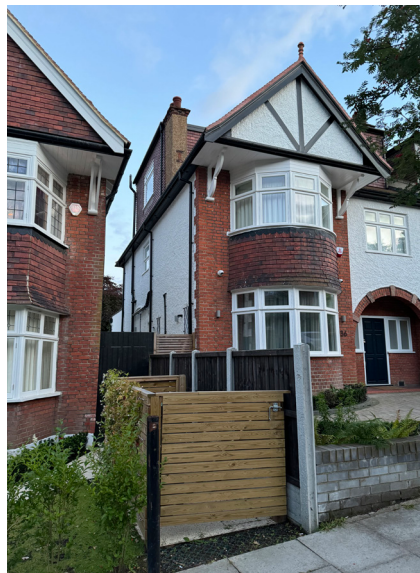
36 Cholmeley Crescent, historic but recently renovated. Significantly larger than the proposal
