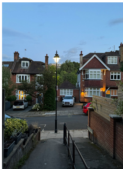
48 & 50 Cholmeley Crescent, historic but
