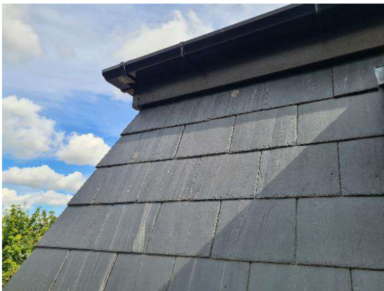
Figure 5: Slate hanging tiles on the rooftop flat, which are all tight-fitting and well-sealed.
