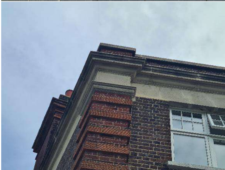
Figure 6: Stone cornicing around the roof verges, which all appears in good condition.
