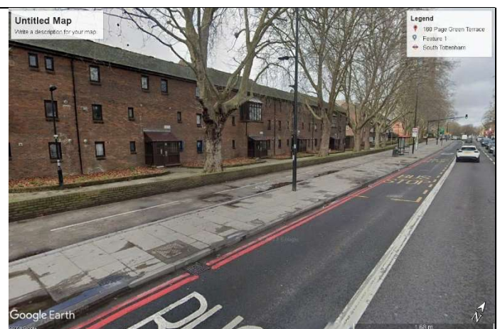
View Looking North West along High Road with the site out of shot to the right
