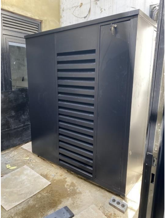
Figure 1– Typical Condenser Attenuated Enclosure
