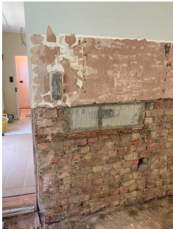
Image 10: opening to be widened – showing some signs of structural problems and open joints.
