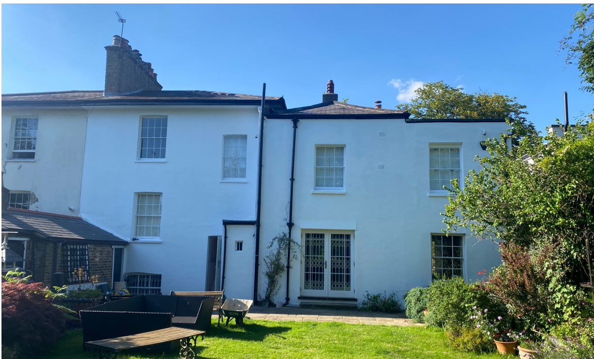
Image 4: S Elevation: flat roof building on E side [right] is formed from a later garage
