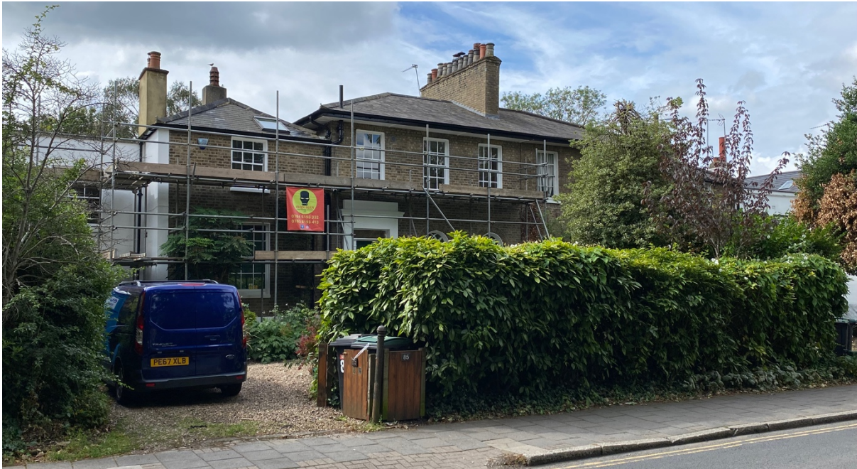
Image 3: N Elevation: lower stucco section on the E side of building (left) is formed from a later garage
