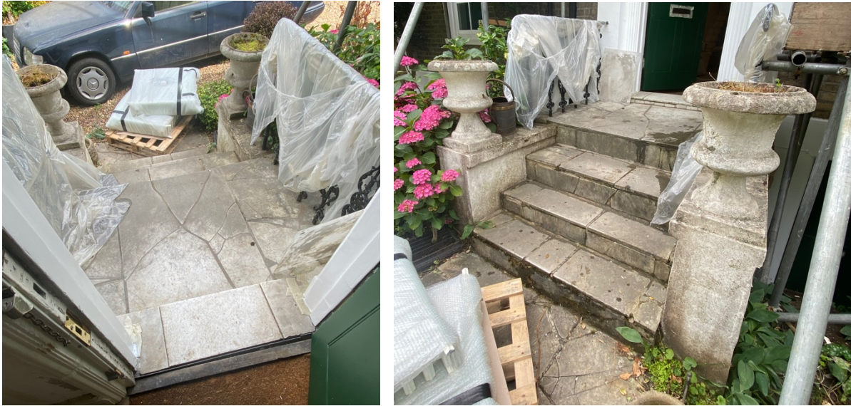
Image 6: New sandstone steps to door to N elevation.
