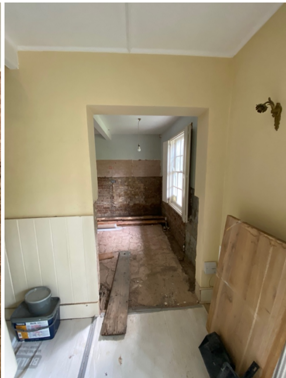
Image 10: opening to be widened – showing some signs of structural problems and open joints.
