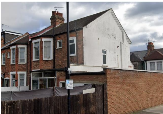
105 Boundary Road – before
