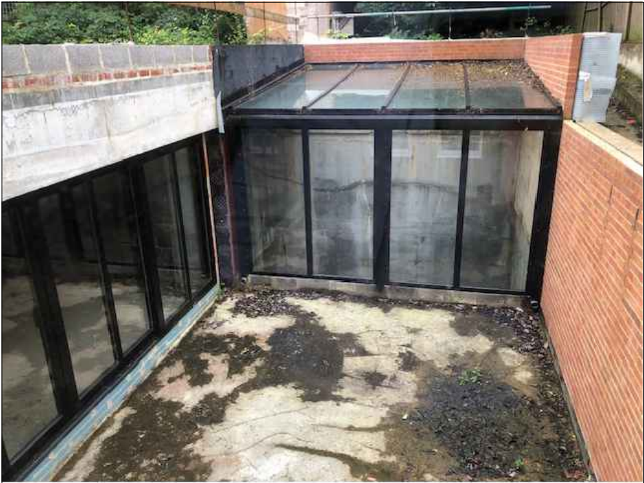
Rear sunken garden
