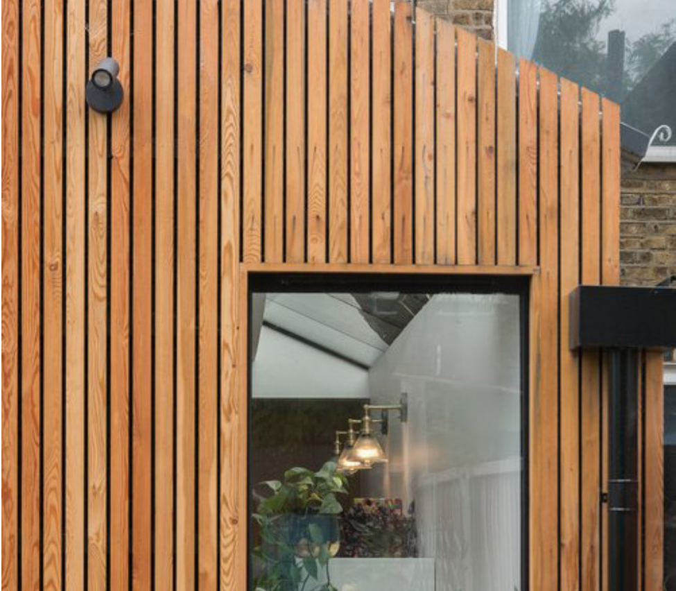
3. Vertical cedar timber cladding battens
