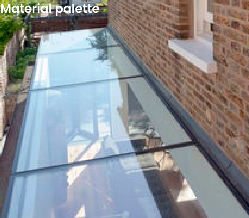
1. Structural roof glazing
