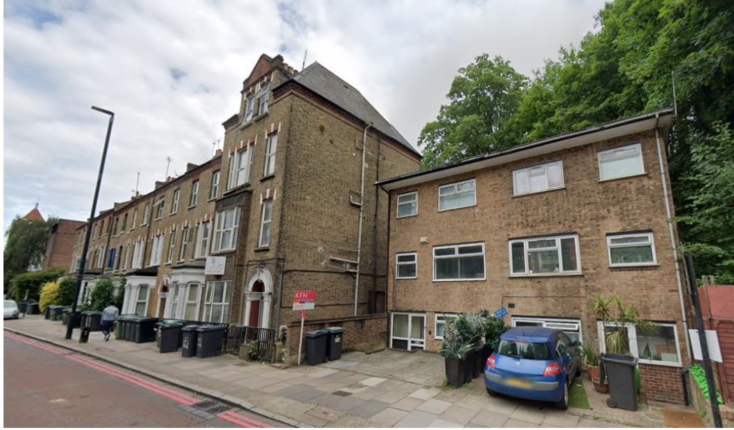
120 ARCHWAY ROAD (SECOND RIGHT) WITHIN THE STREET SCENE
