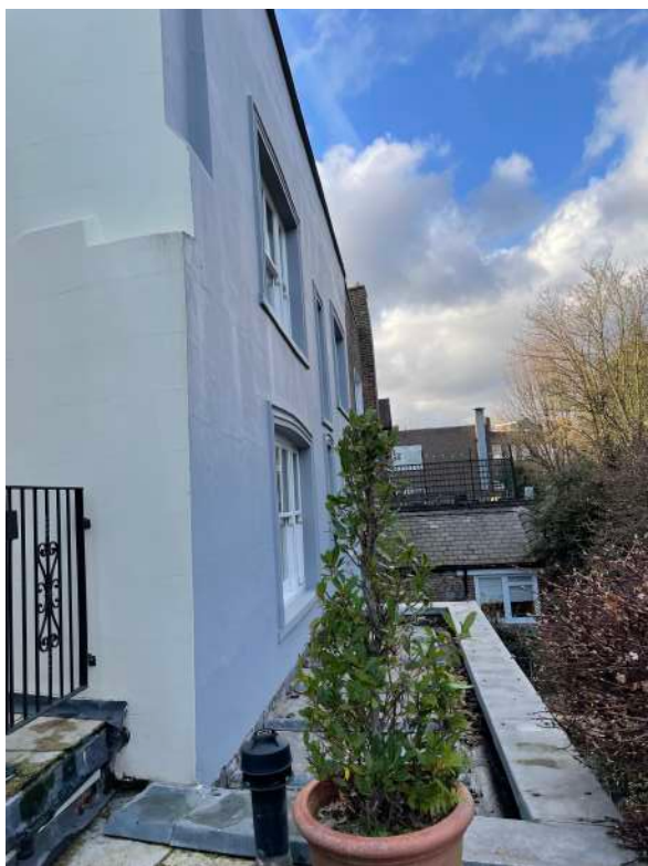
View of rear extension to No.94
