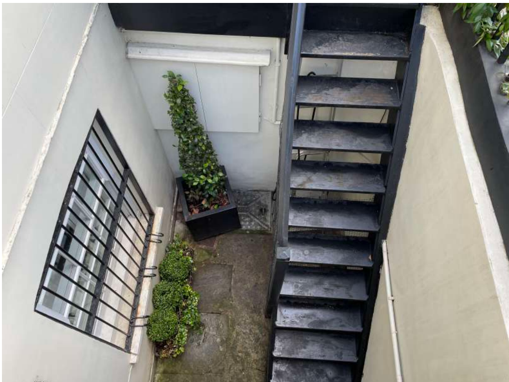
View of stair in front lightwell leading to Basement
