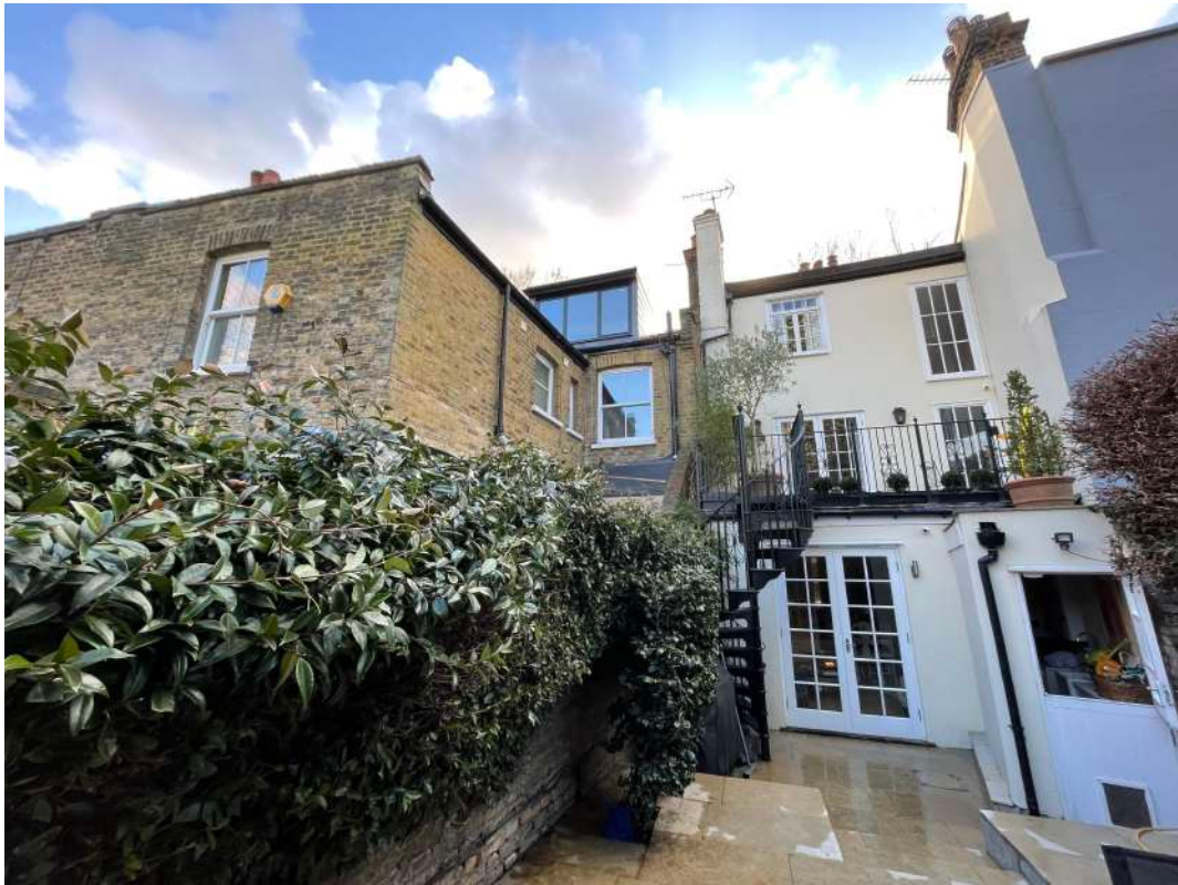
Existing rear view of No.90 on LHS & No.92 on RHS
