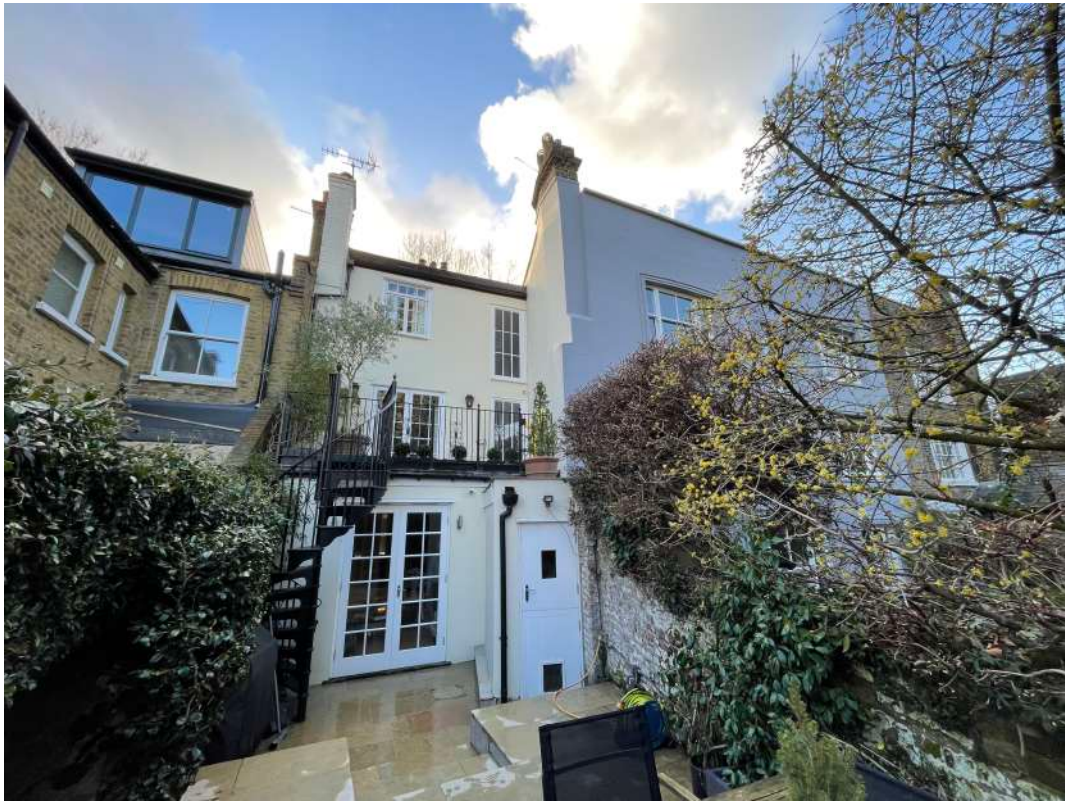
Existing rear view with No.92 centre. No. 90 on LHS & No. 94 on RHS
