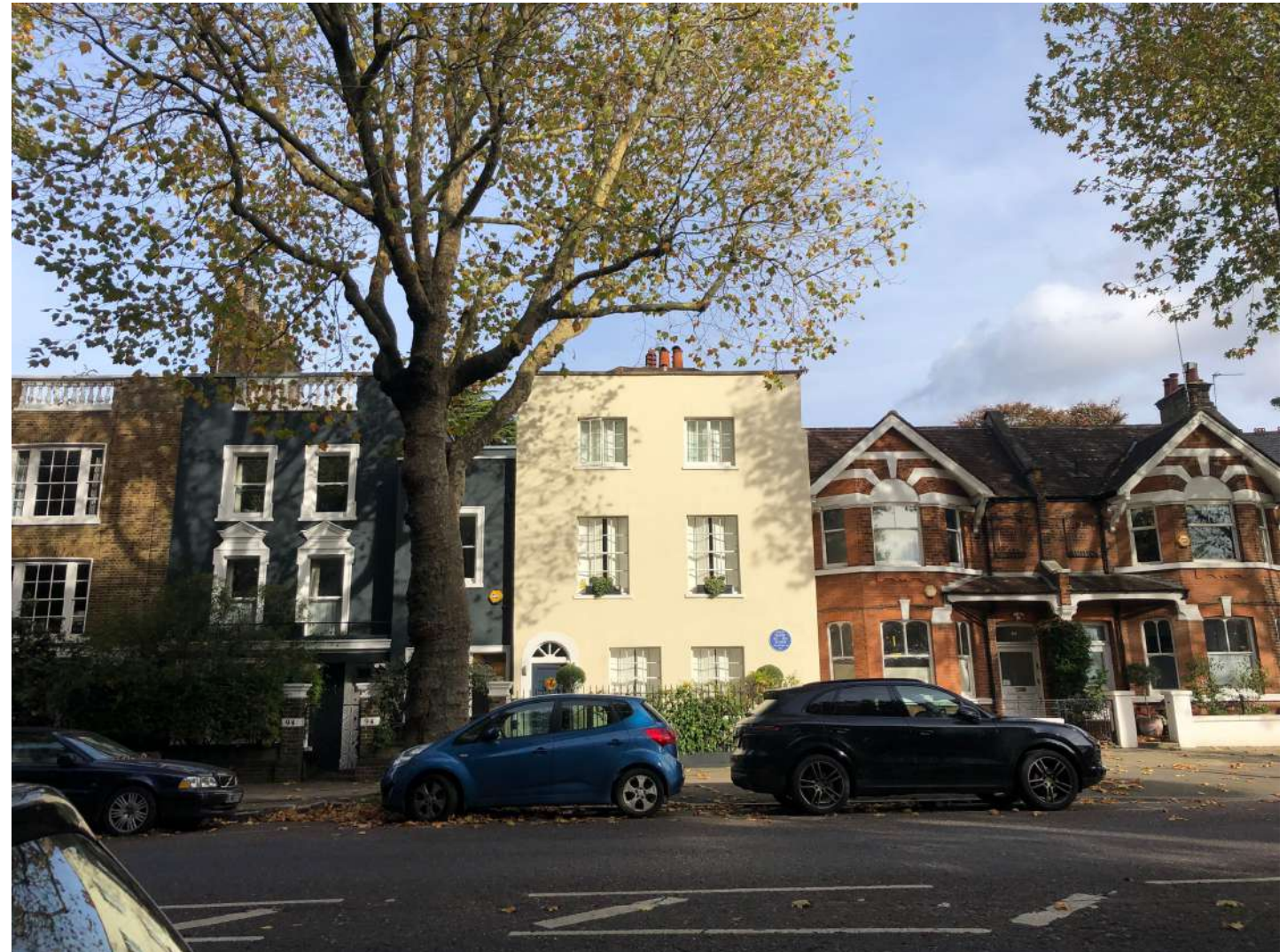
Front elevation showing No. 92 North Road centre, off white render, with No. 90 on RHS & No. 94 on LHS
