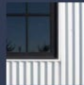
Profiled metal balcony cladding
