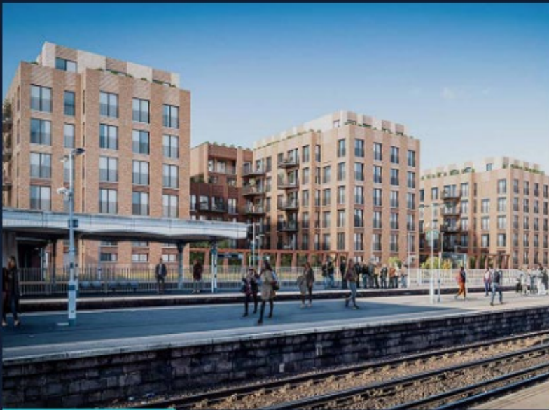
Purley Station car park by J Group
