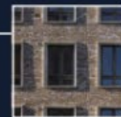
Metal window with projecting surrounds
