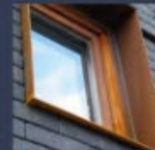
Metal window with projecting surrounds
