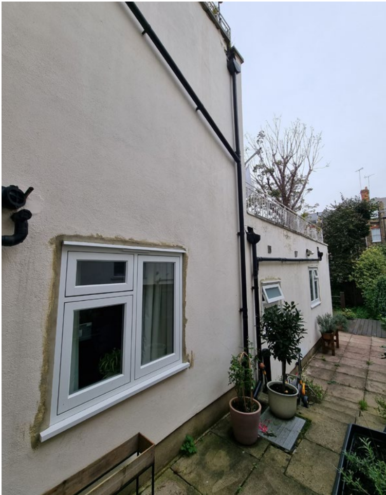
View to outrigger elevation from side alley at Flat A
