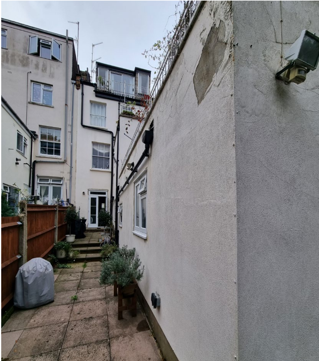
View to outrigger elevation from side alley at Flat A
