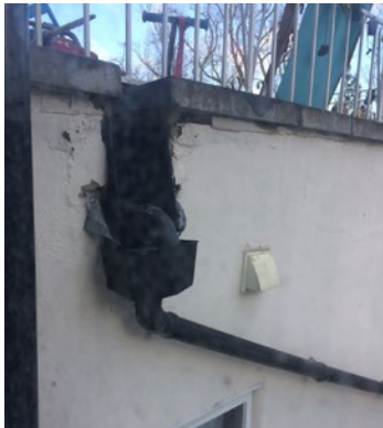
View to hopper serving serving surface water drainage from Flat C terrace
