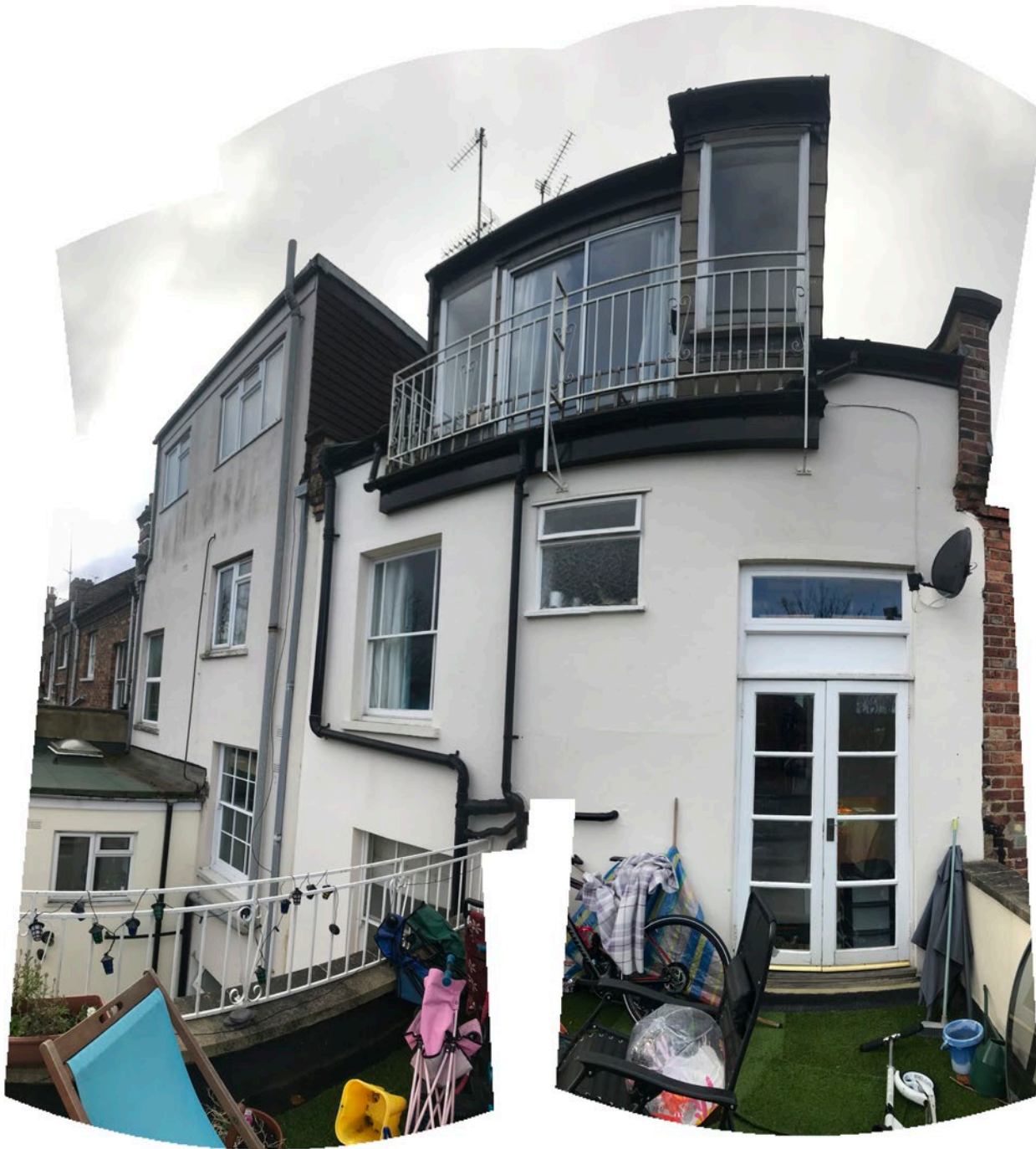
View from terrace at Flat C to rear elevation
