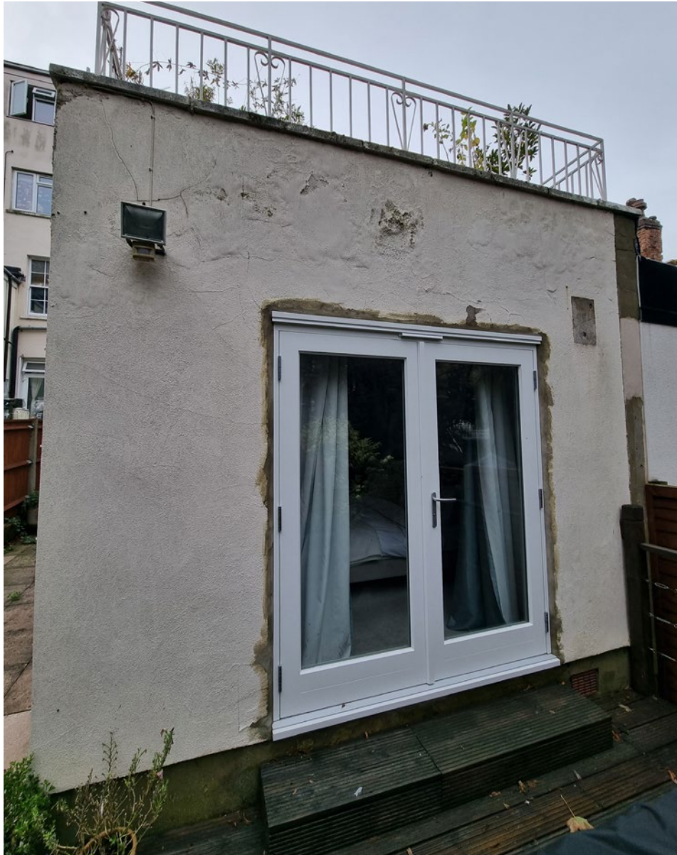
View to rear elevation of extension at rear of Flat A
