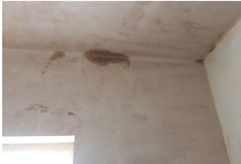
Damage to ceilings below roof terraces
