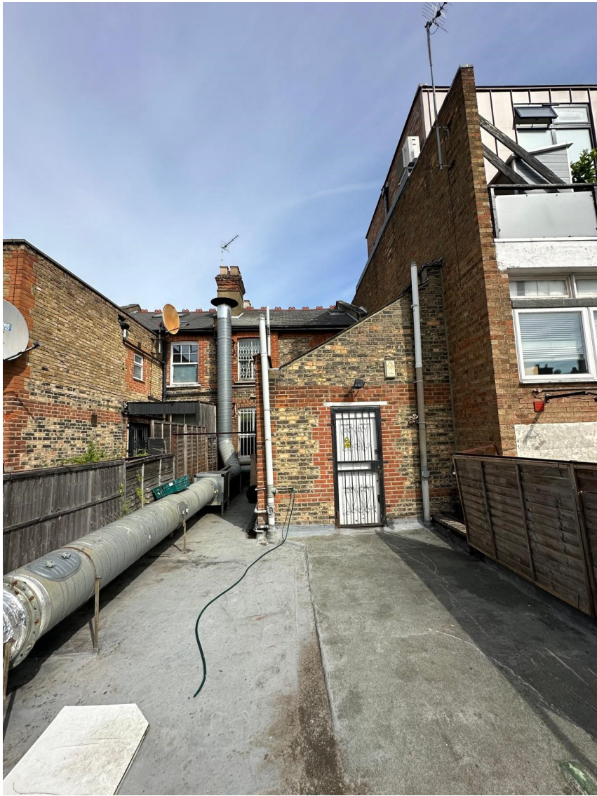
• Existing Extension View •
