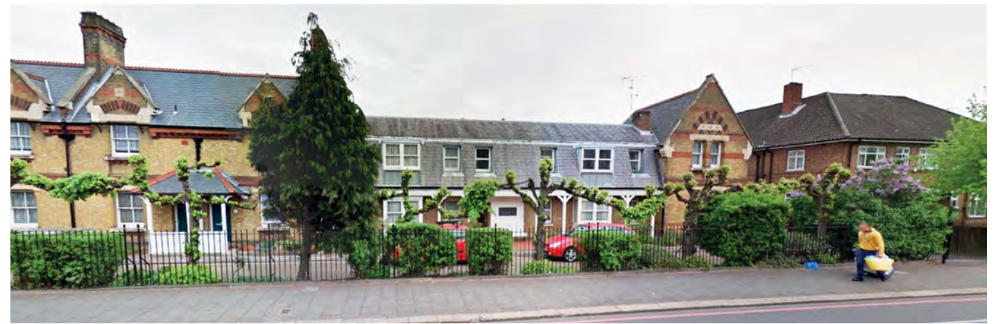
VIEW 2 - VIEW OF THE 1970'S INFILL BUILDING
