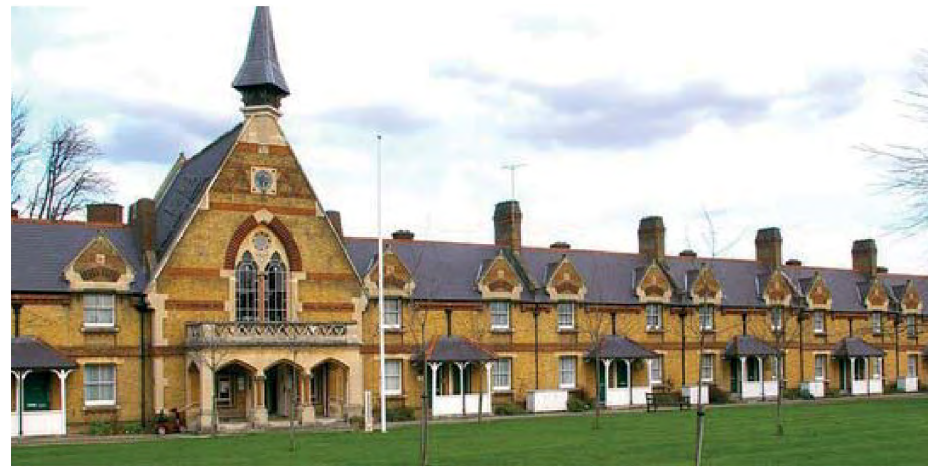
VIEW 1 - VIEW OF THE CENTRAL FORMER CHAPEL
