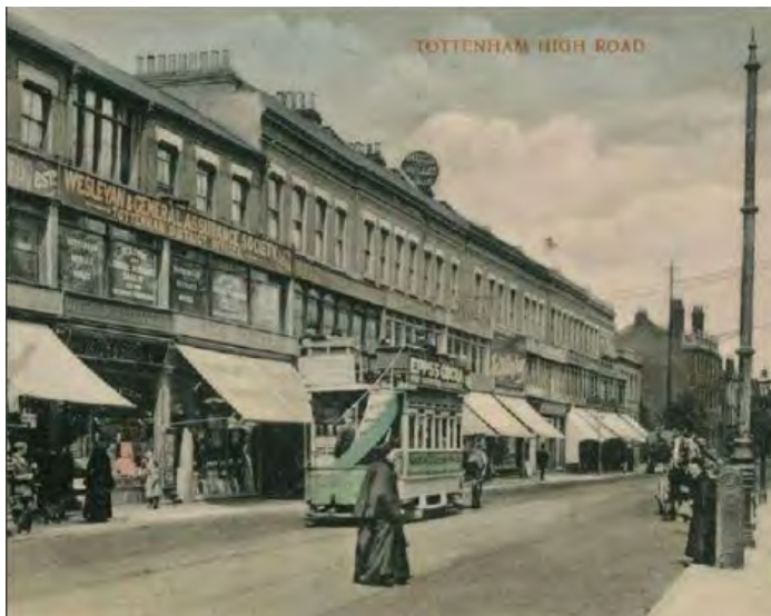
HISTORIC PHOTOGRAPH LOOKING NORTH FROM BRUCE GROVE STATION (TAKEN FROM HARINGEY WEBSITE)
