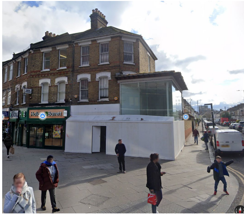
View from High Road
