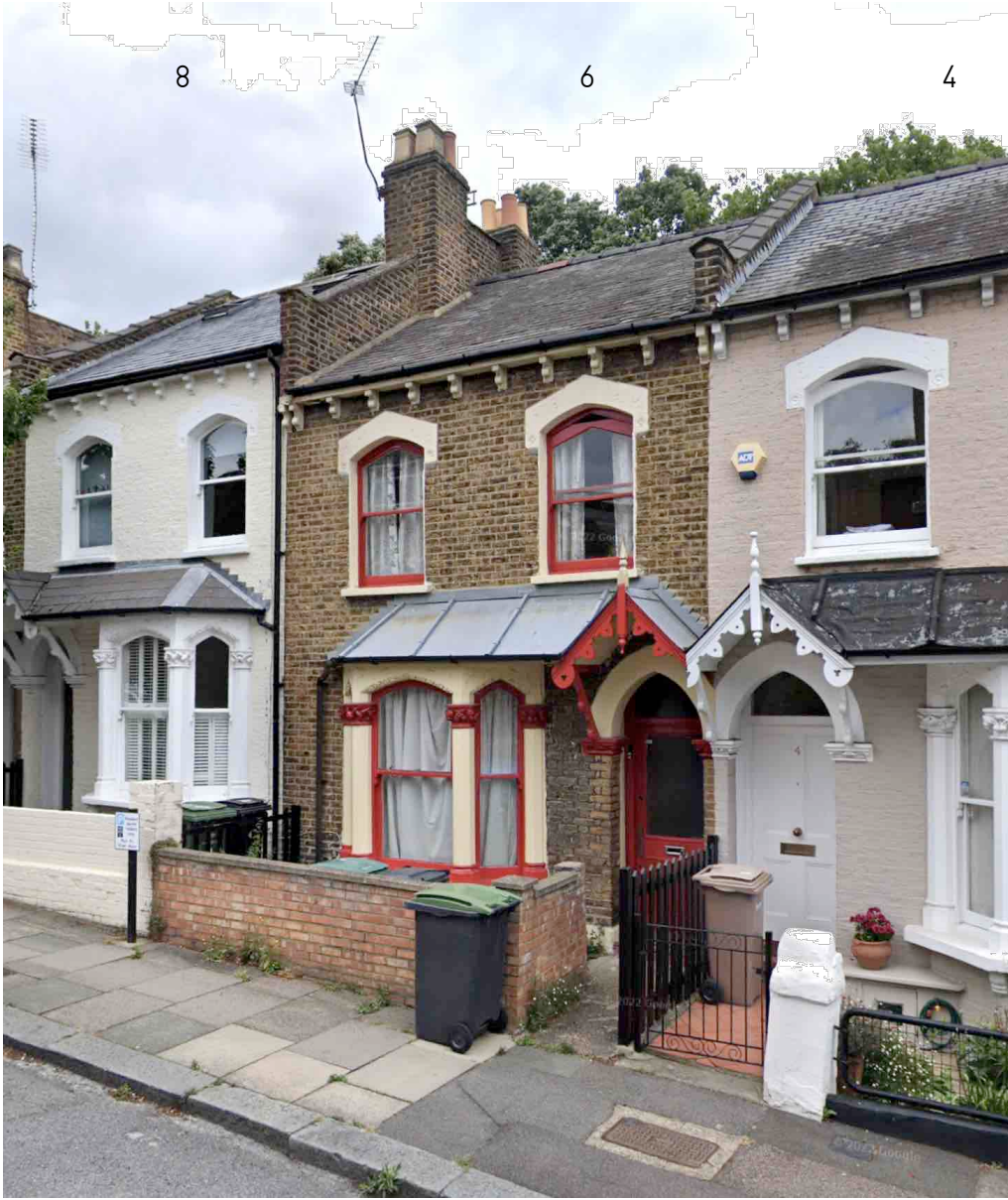
Existing Orchard Road Facade
