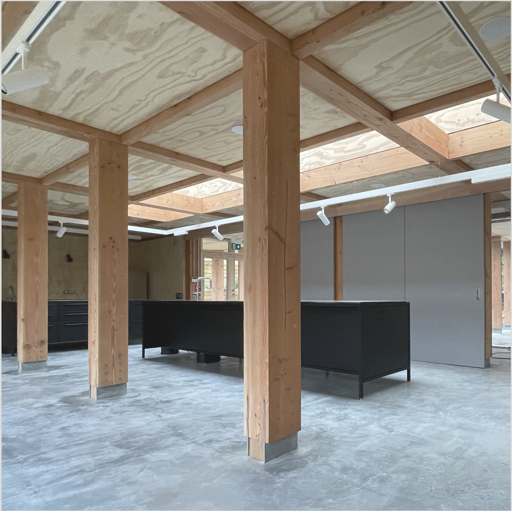
Structural Frame - Solid timber structural framing/cladding with clear finish
