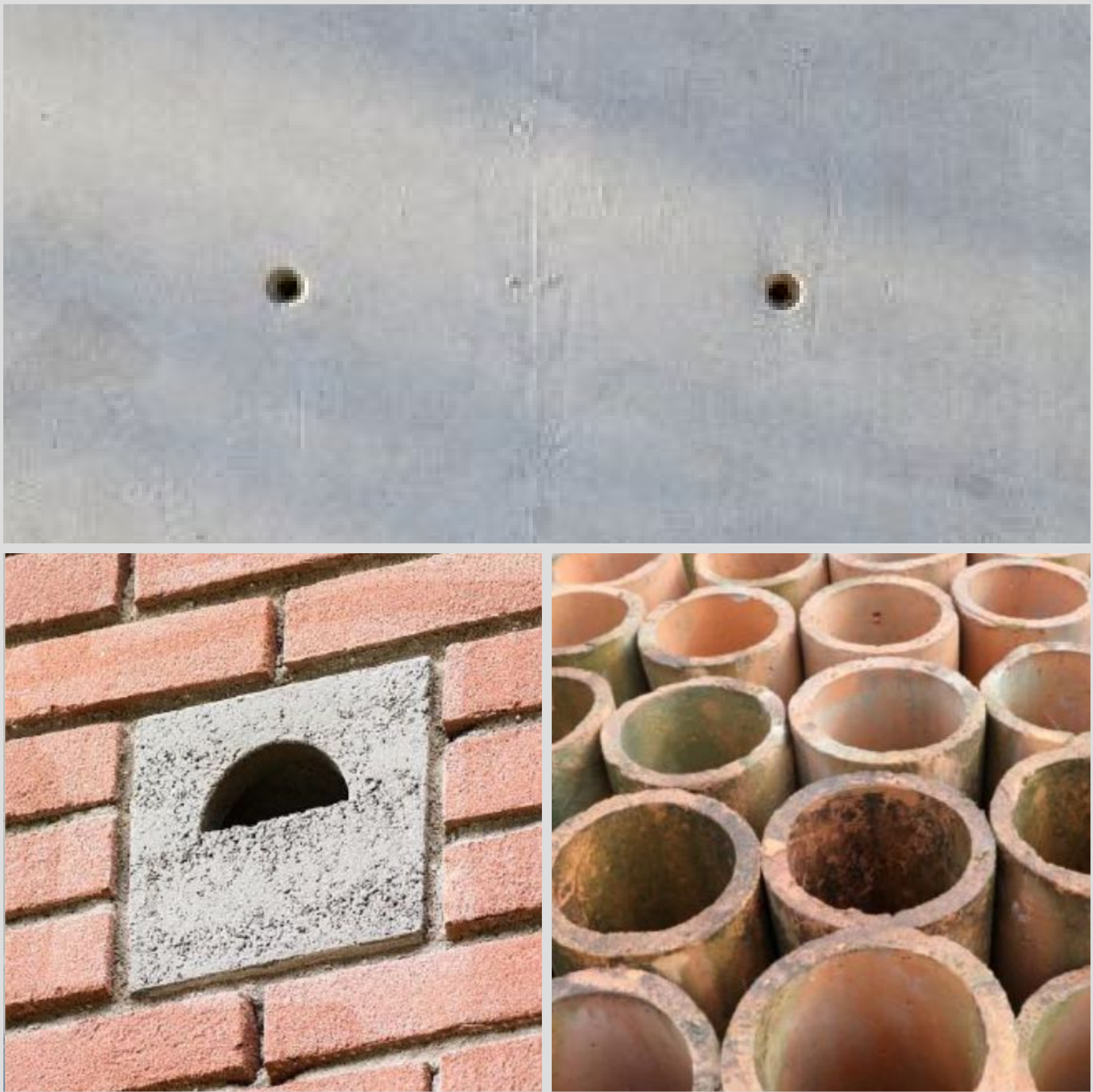
Walls - Fairfaced concrete walls Wall Lining - Brickwork/blockwork/tile wall lining
