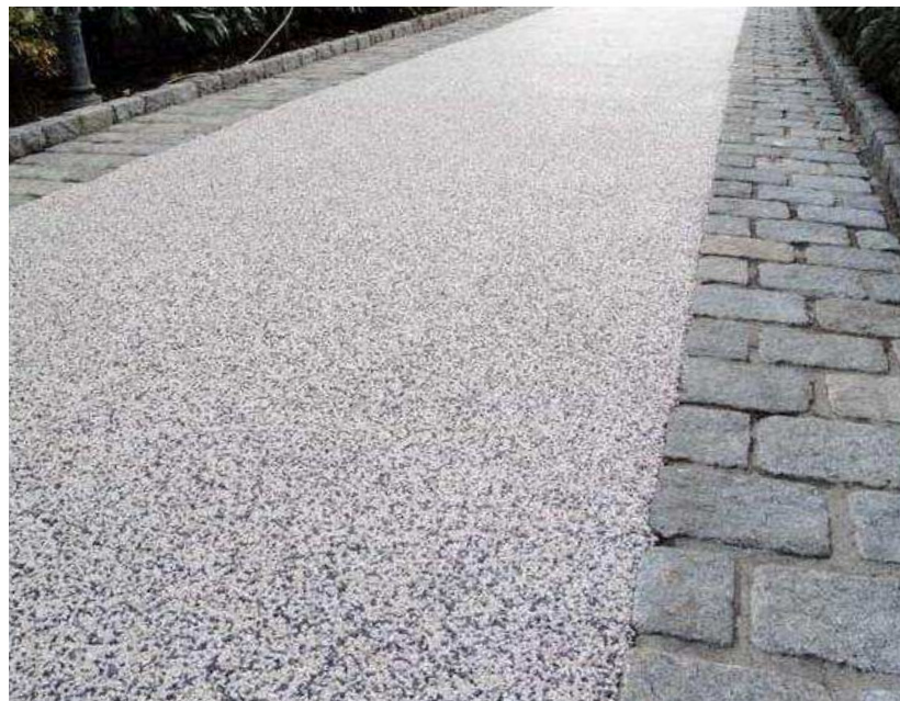
Example of resin bound gravel pavement with granite sett border
