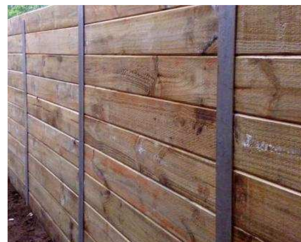
Reinforced hardwood sleeper retaining wall
