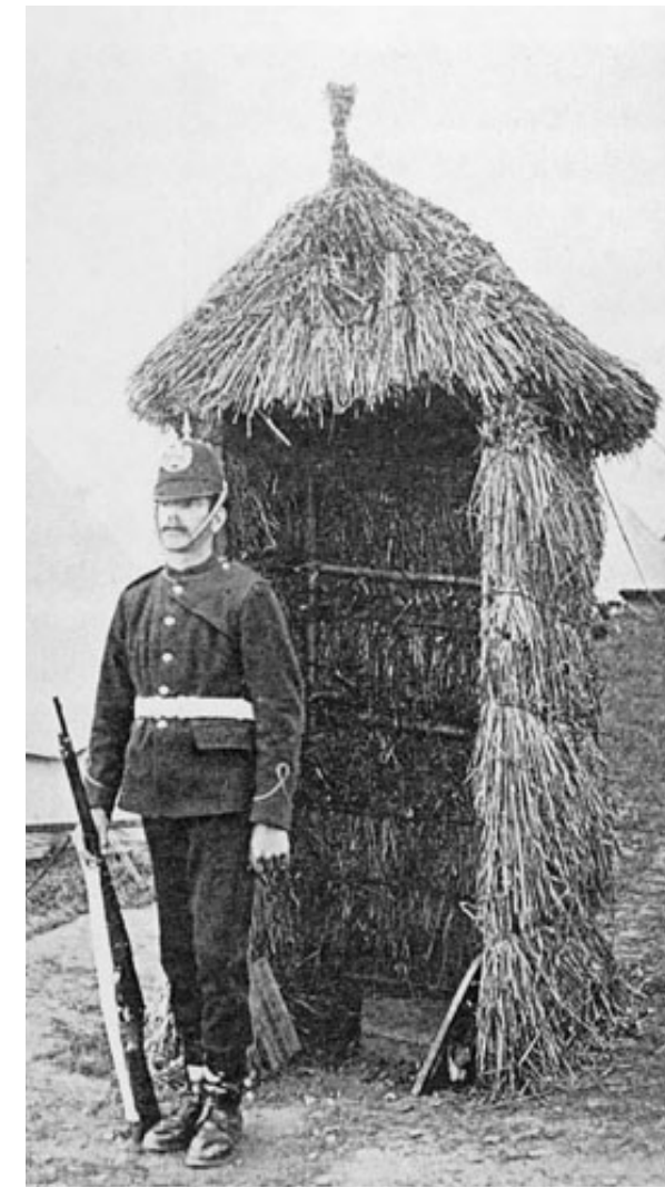
Historic example of rudimentary guardhouse
