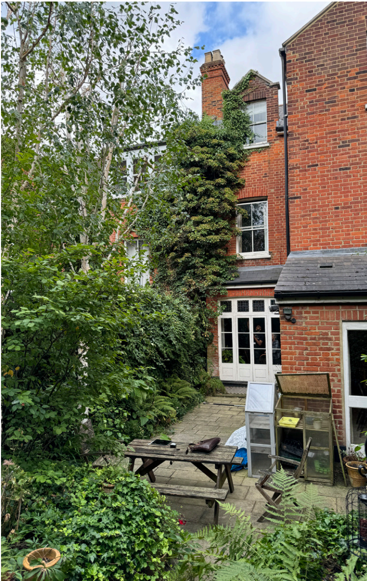
Boundary with 56 Cromwell Avenue at rear
