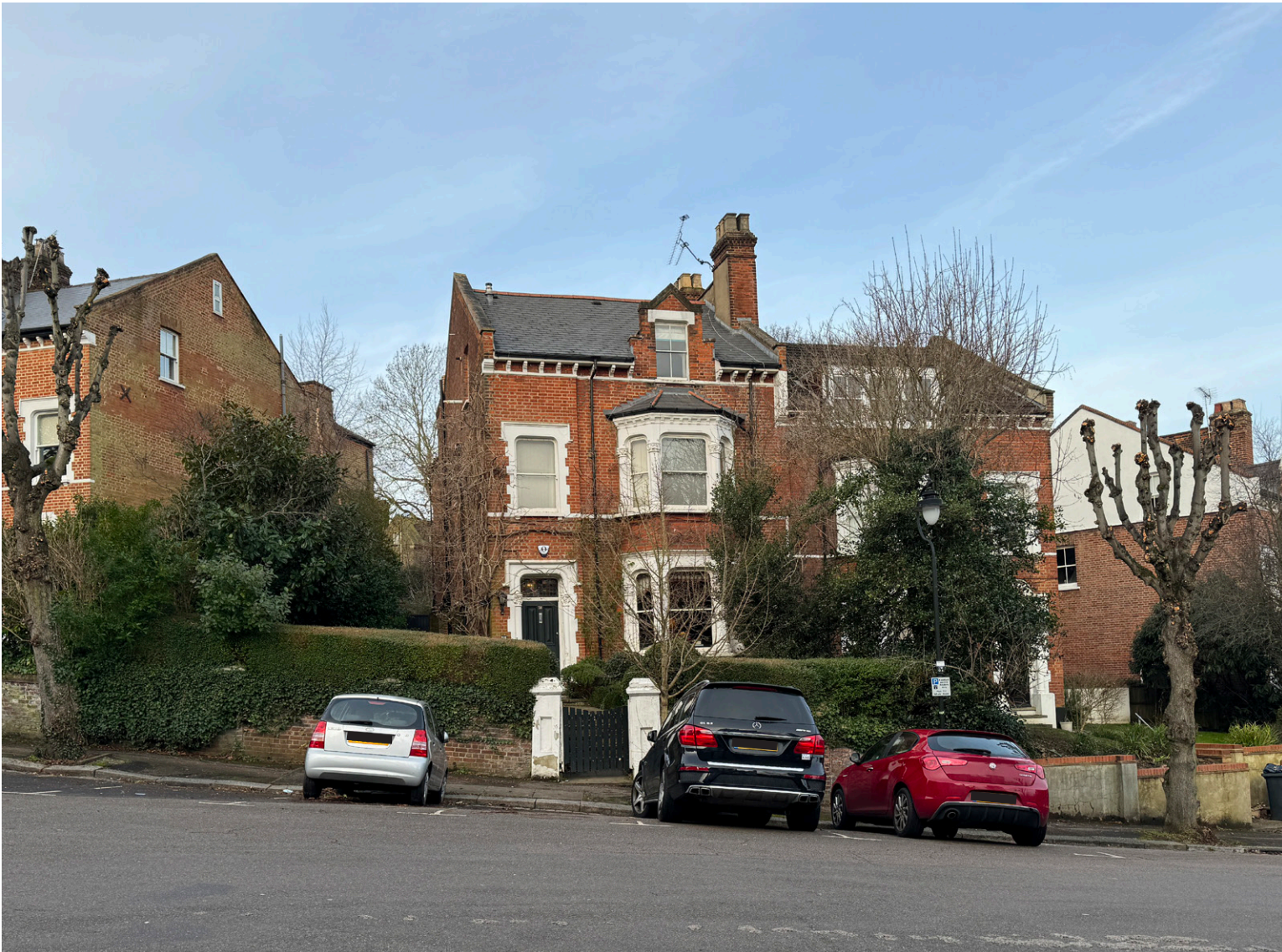
Front (South) Street Elevation
