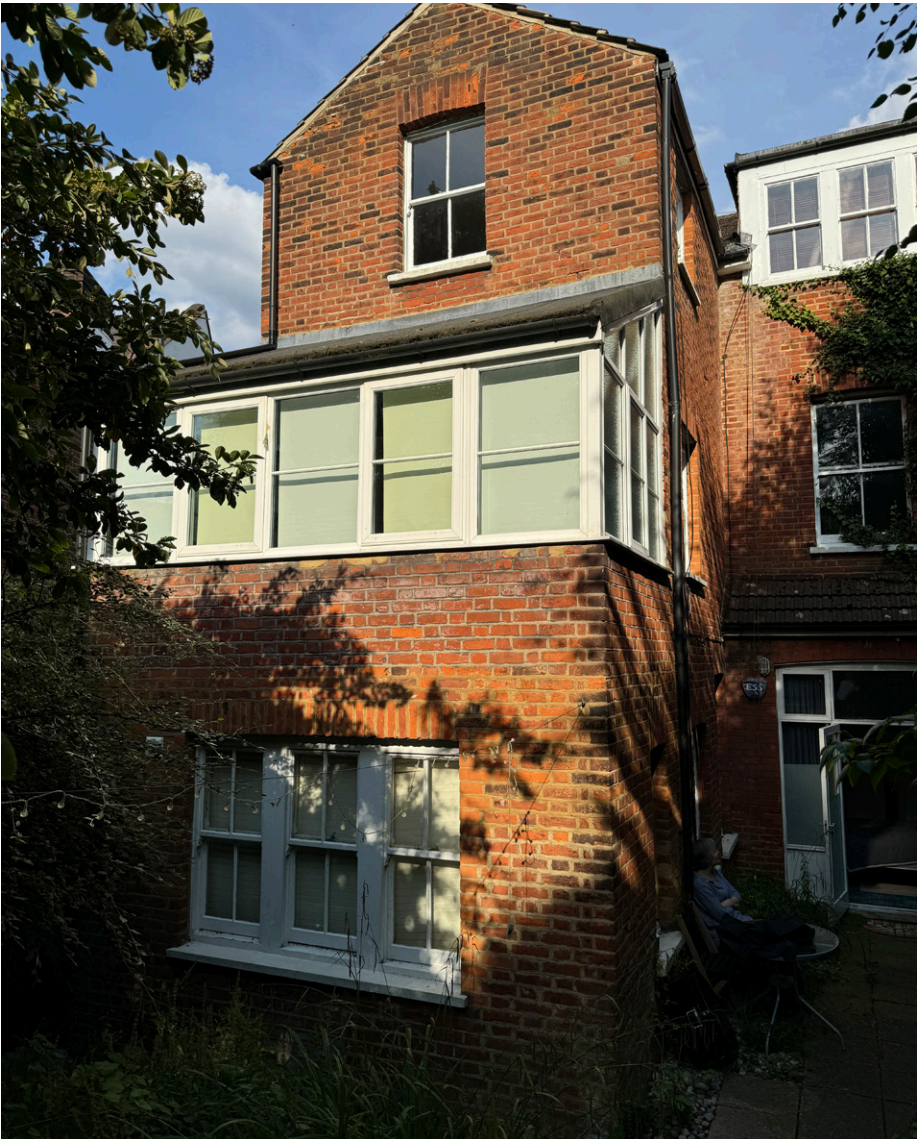
Extension to rear of 56 Cromwell Avenue
