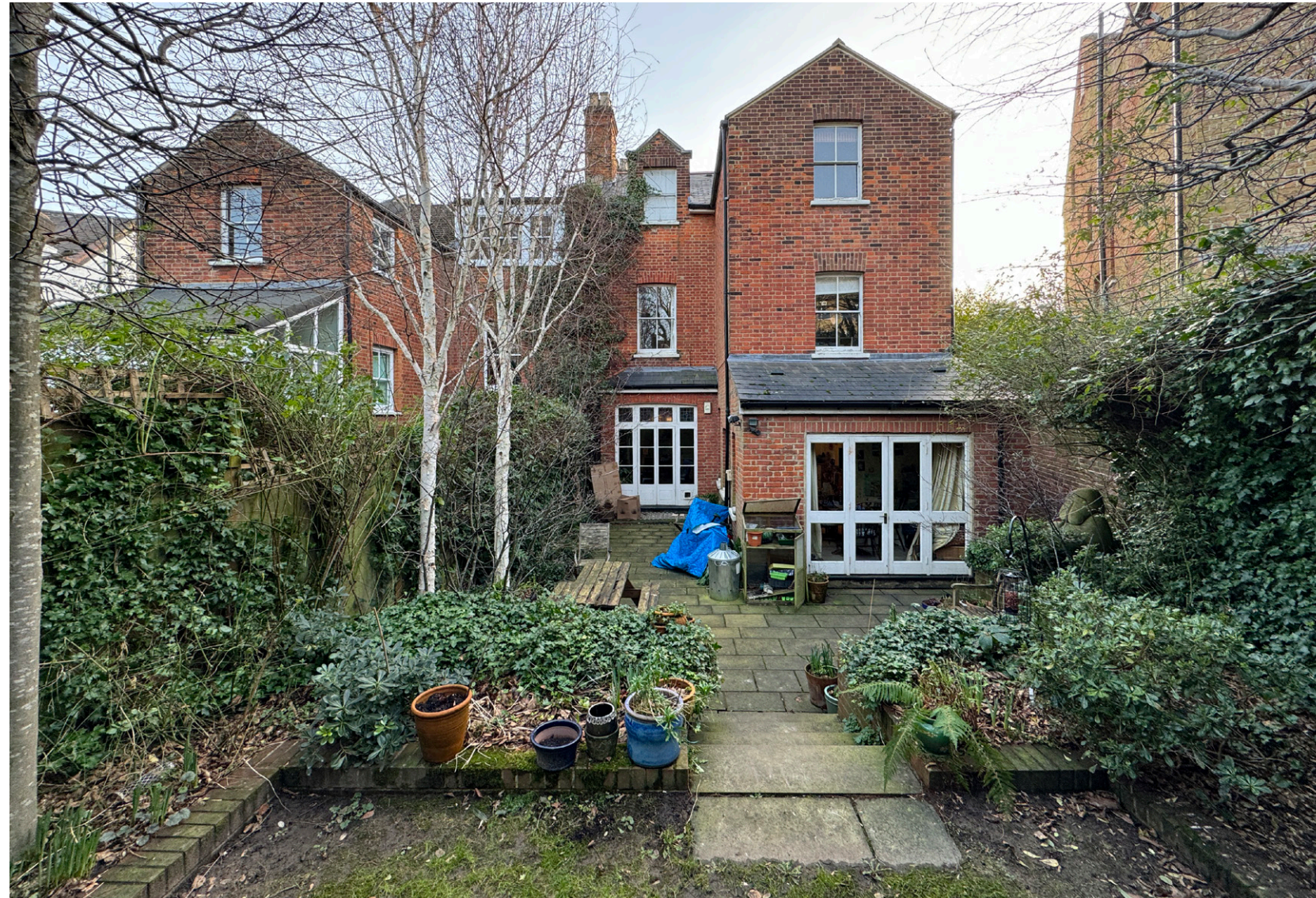
Rear Elevation - Wide View
