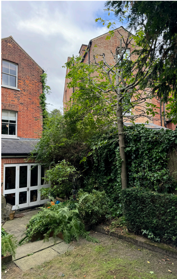
Boundary with 60 Cromwell Avenue at rear
