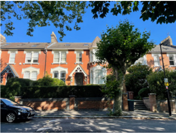
a. front of host building from street
