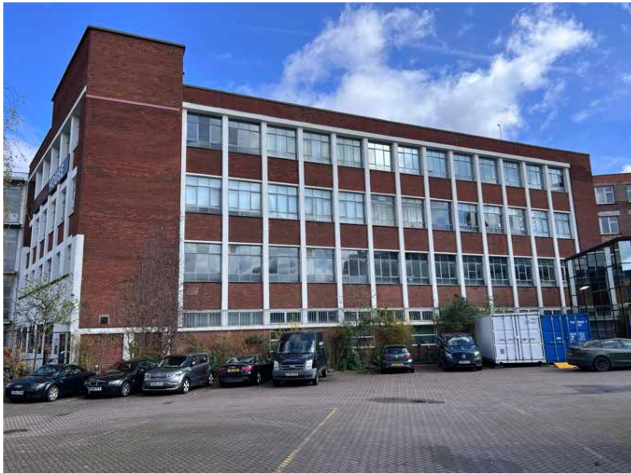
South Facade from adjacent car park
