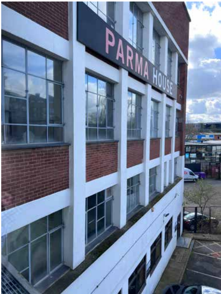
West facade from lightwell
