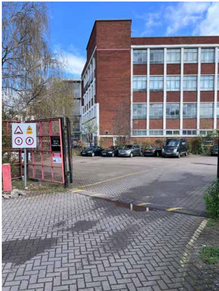
Recently completed 'Vabel' scheme to the south, rear courtyard
