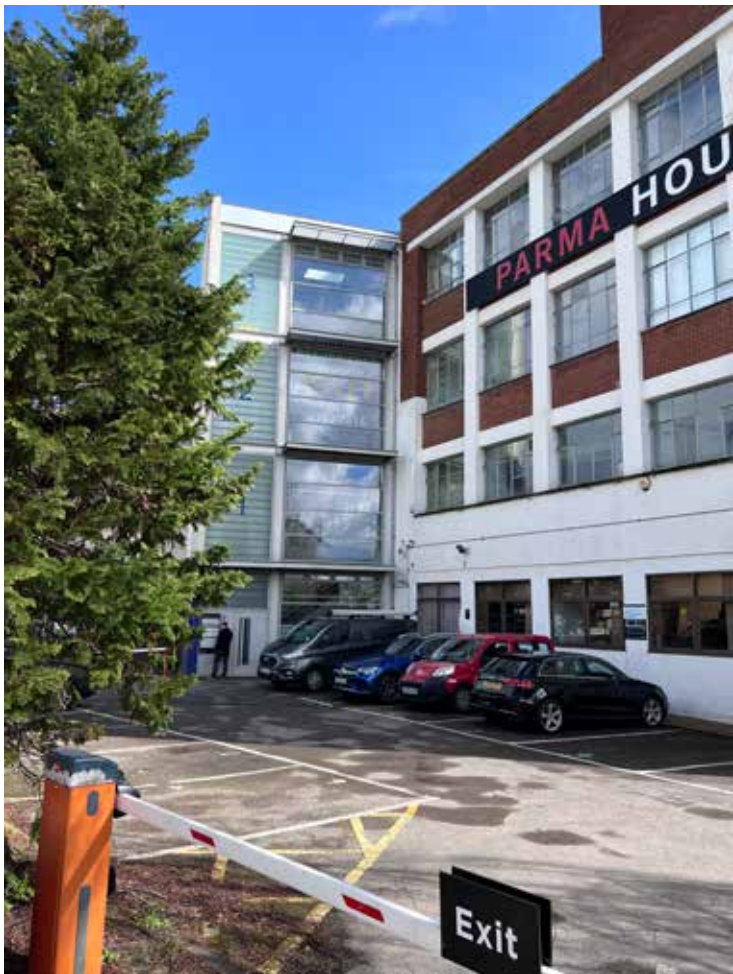
West facade from lightwell
