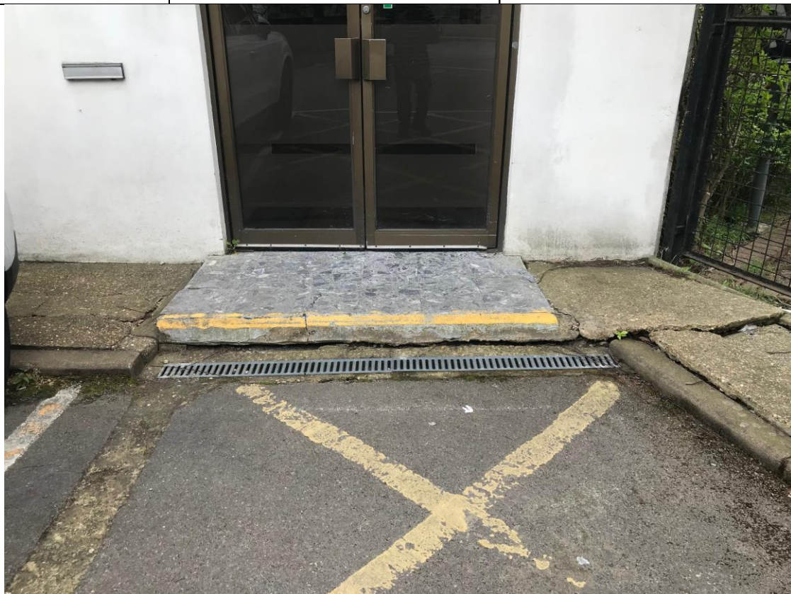
Photo 6: Gully channel drains noted at the building entrance
