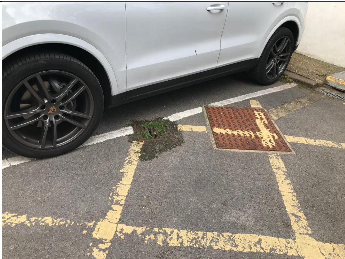
Photo 5: Manhole and drain were noted in the car park
