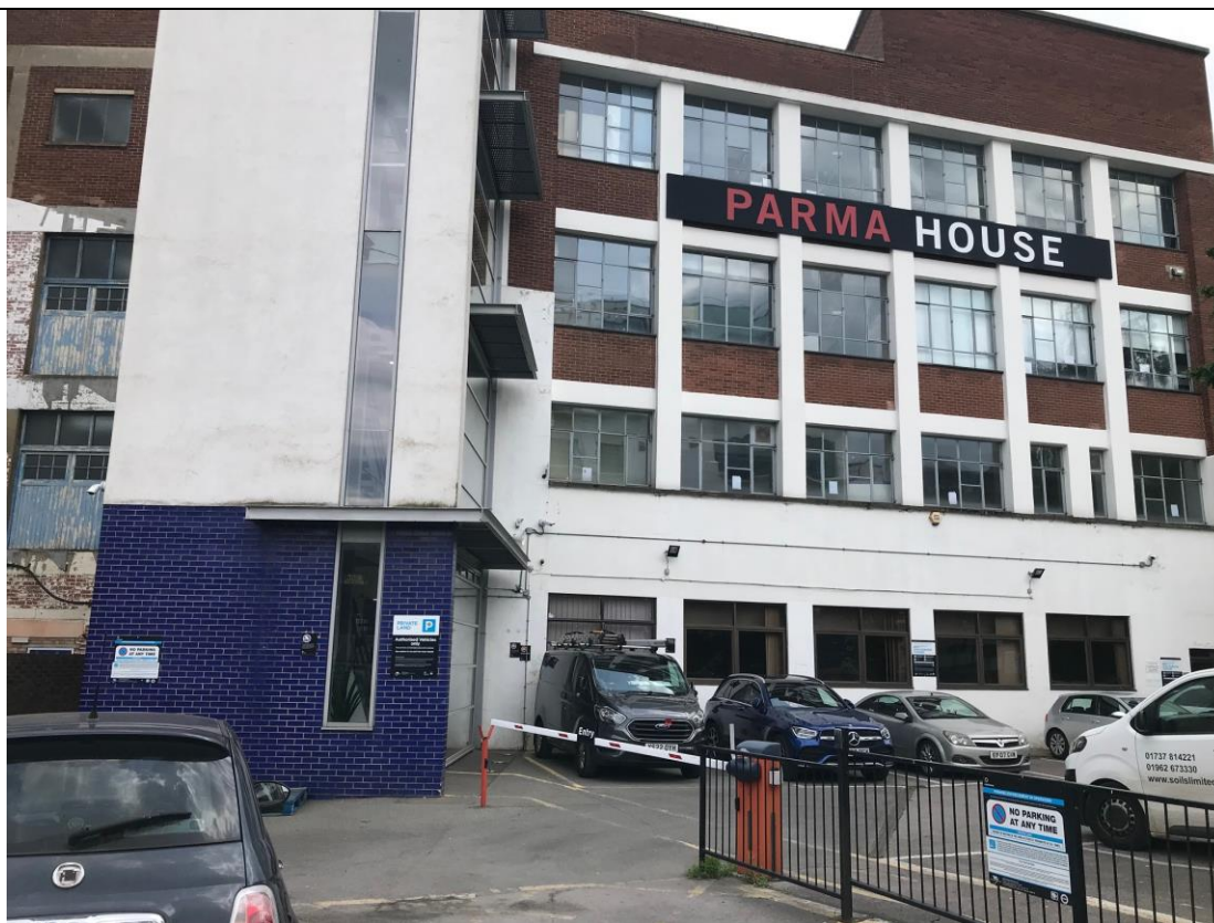
Photo 1: Front of the building with car park
