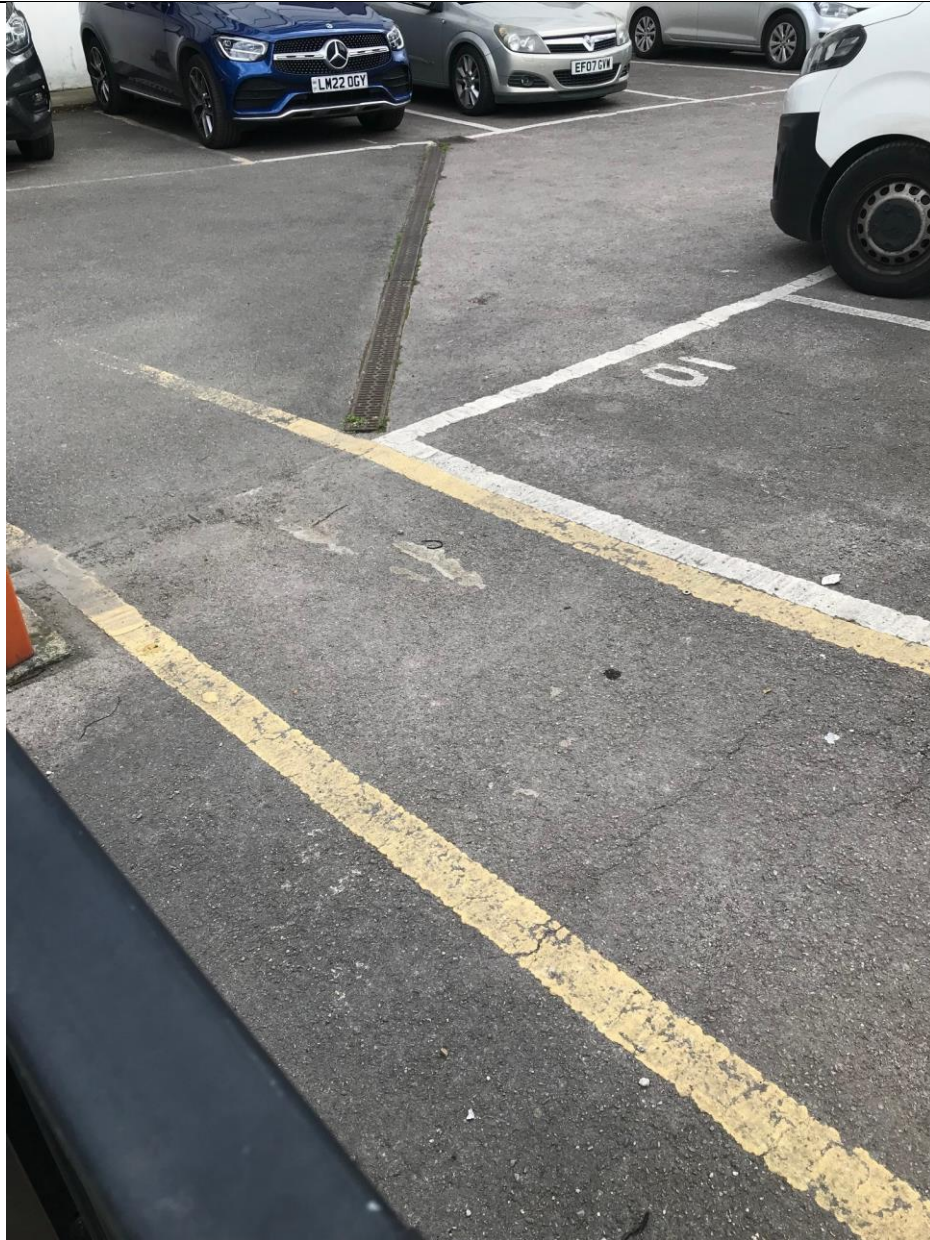
Photo 7: Gully channel drains noted onsite
