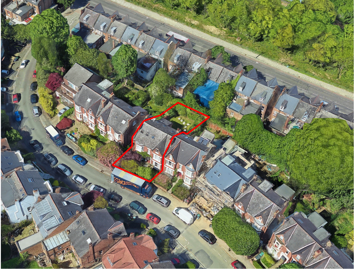
fig.1 aerial photography, google maps - no. 67 Talbot Road outlined in red
