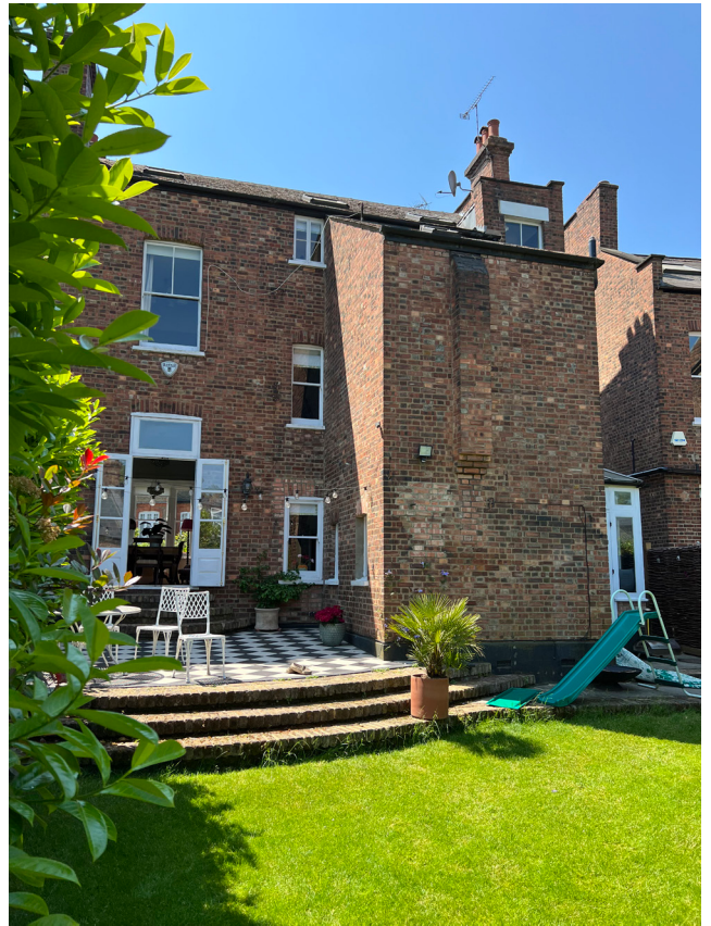
fig. 3 rear view of no. 67 showing two storey existing outrigger
