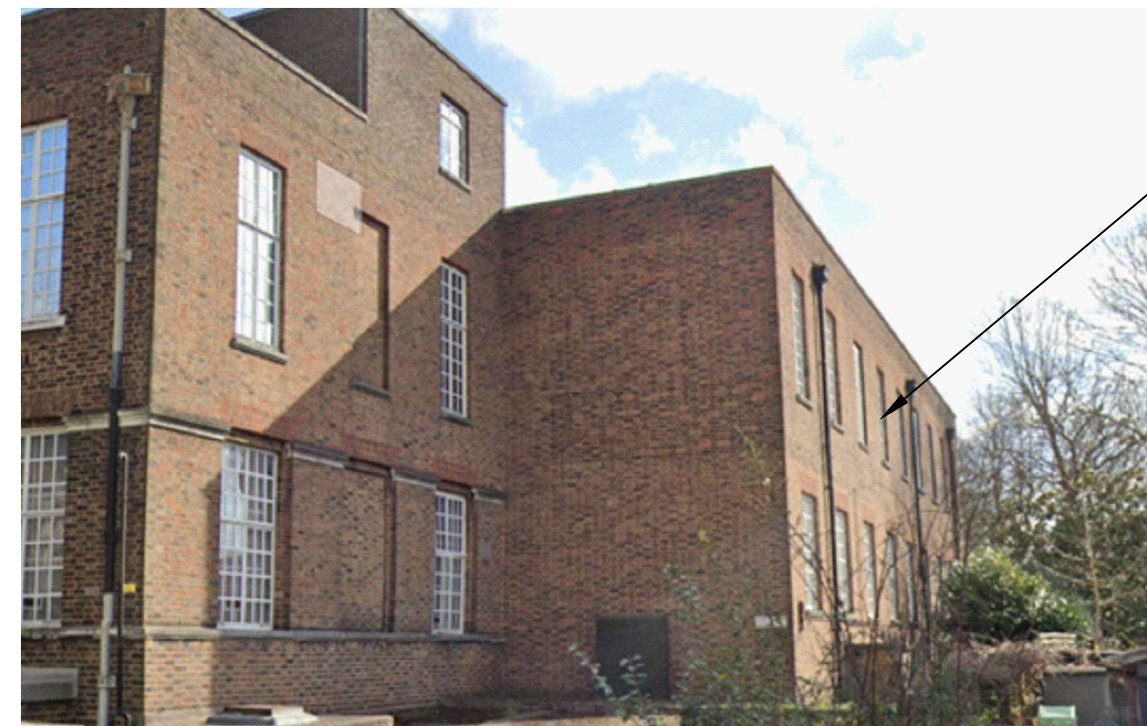
PHOTO OF WEST ELEVATION
