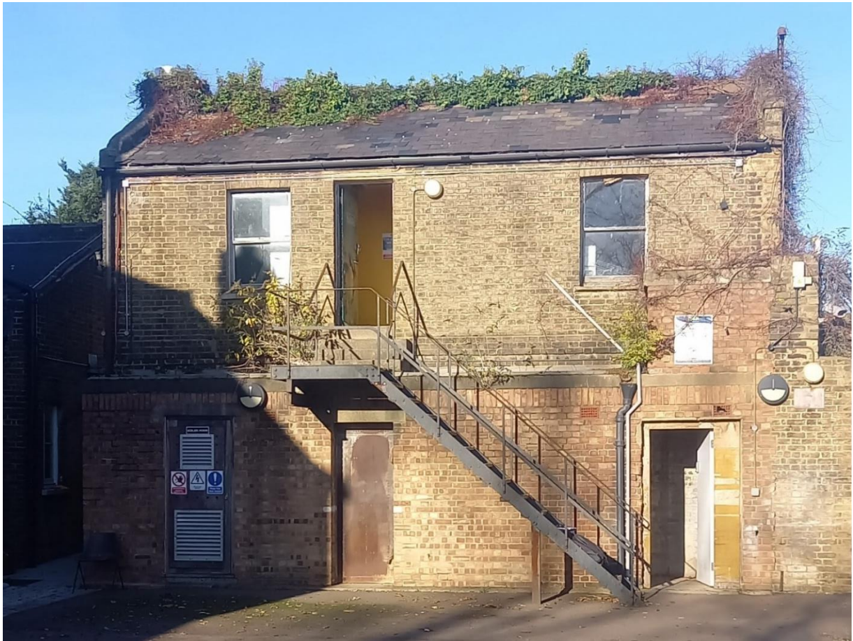
View from car park (South Elevation)
