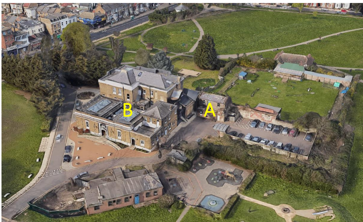
Aerial view of Woodside Park (Annexe [A] George Meehan House [B])
