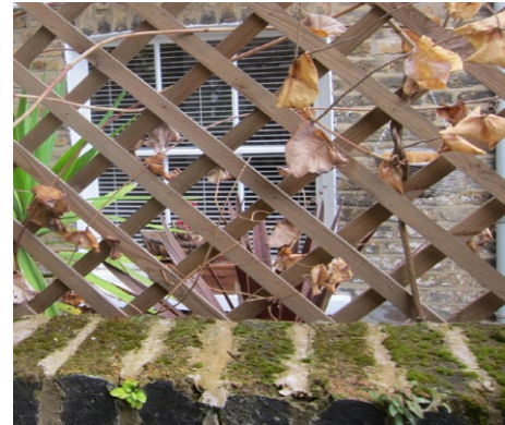
Neighbours trellising above masonry boundary wall for privacy.
