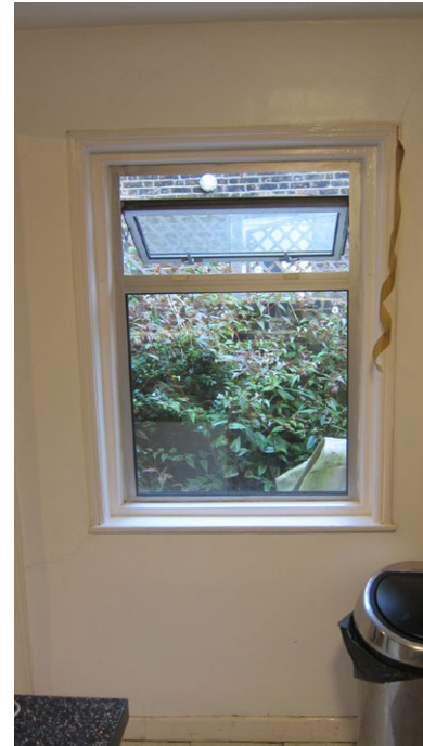
Kitchen window facing directly onto neighbours window
