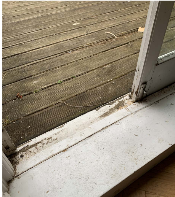
Figure 12. Photograph of the existing patio decking and patio door.
