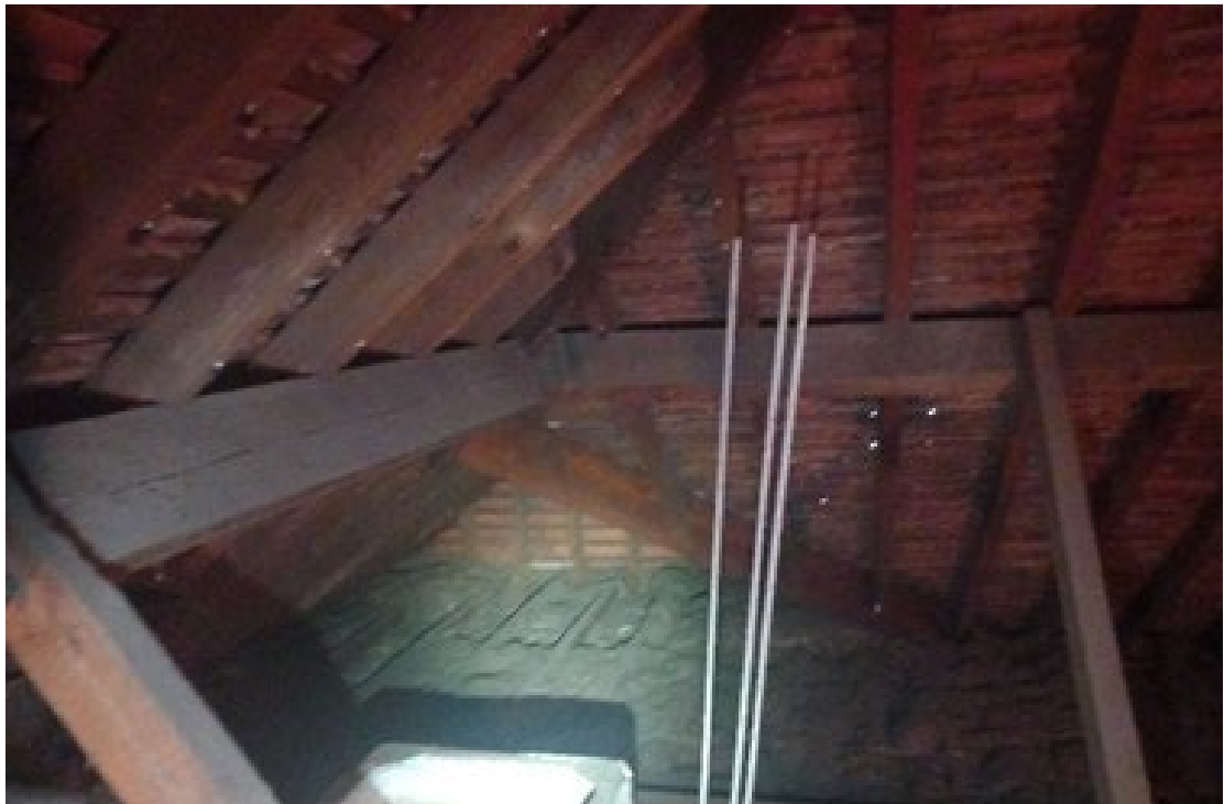
Photo 3 - Building 1 - Interior loft void
