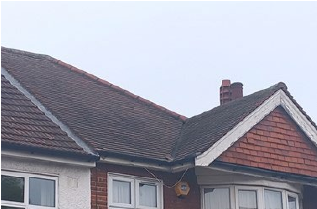
Photo 6 - Building 1 - Front tiles and hung tiles
