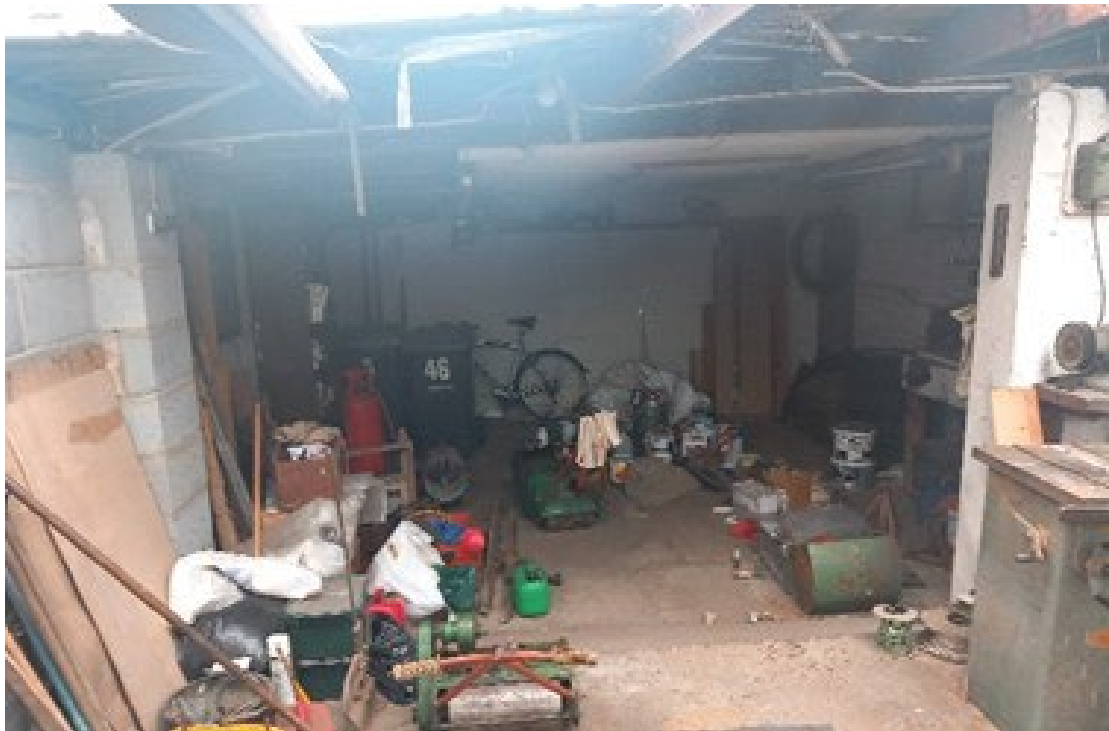
Photo 14 - Building 4 - Western interior
