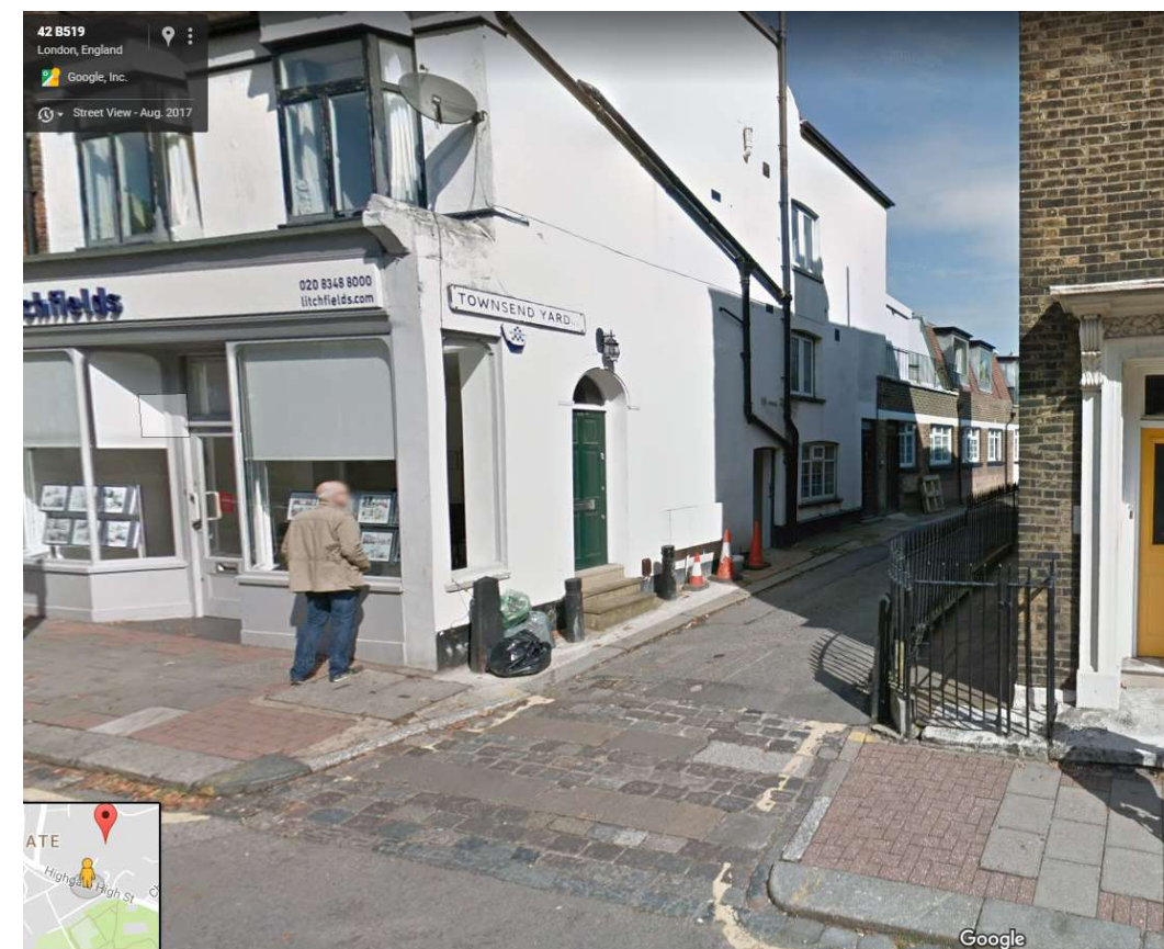
Figure 5 – Confined site access from Highgate High Street
