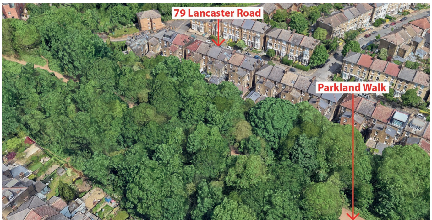
Figure 03 - Aerial photograph of Parkland Walk and 79 Lancaster Road
