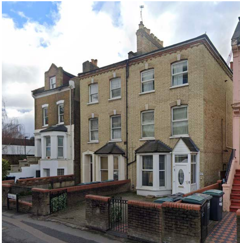
01. View of front (North) elevation and public footpath (looking south east)
