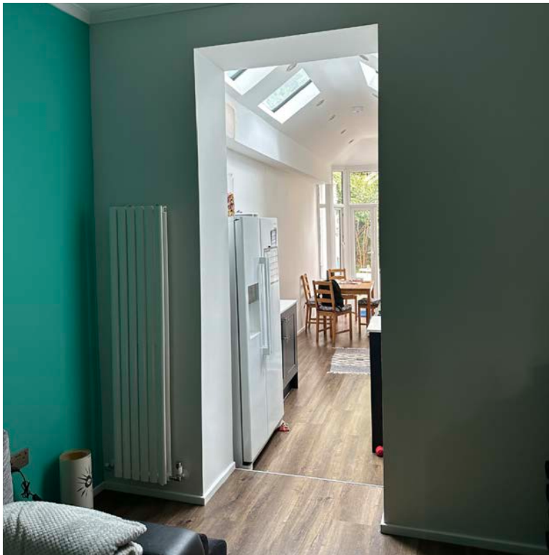
02. View of existing lounge area
