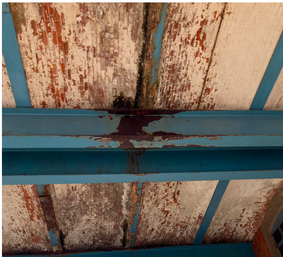
Figure 9: Beams and vaulted brickwork
