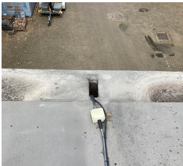
Figure 4: Existing Rainwater outlet into Cast Iron column
