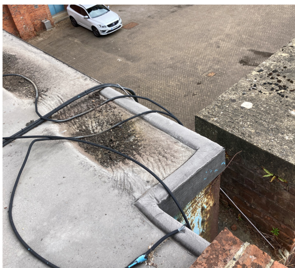
Figure 6: Blistered asphalt either side of bridge
