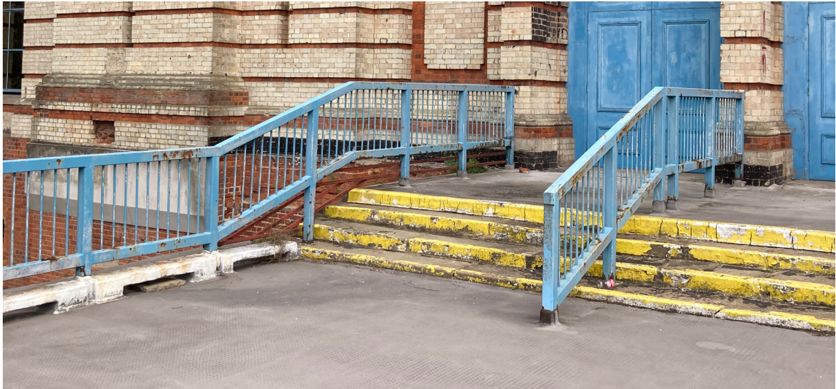
Figure 1: Existing entrance to Great Hall including asphalt covering, stone steps and metal balustrade
