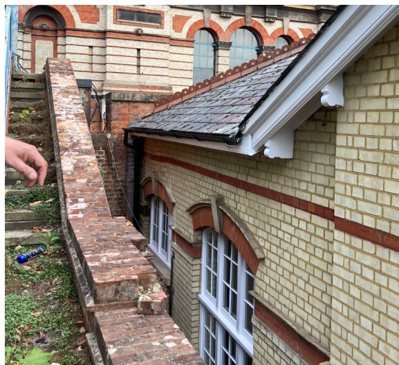
Figure 5: Brick wall to lower steps
