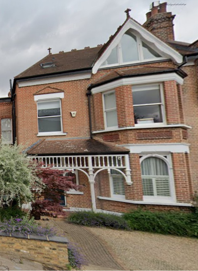
03. Neighbouring Property along Southwood Ave.
