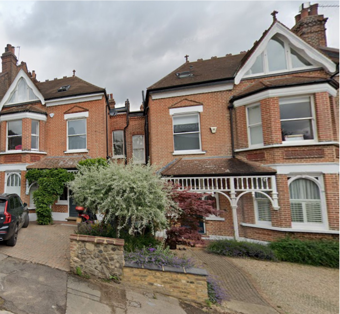
Above: Photograph of typical properties along Southwood Avenue, N6.
