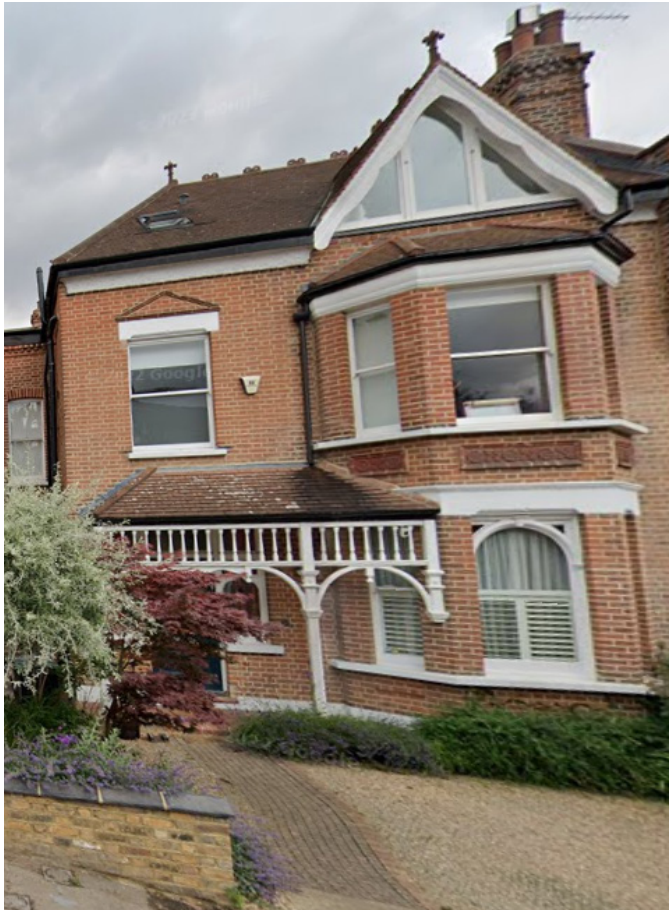
03. Neighbouring Property along Southwood Ave.
