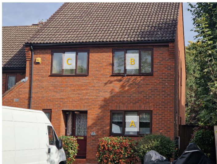
Figure 3 Windows at 4 Jacqueline Creft Terrace, Grange Road. This property was analysed using the obstruction angle criterion.
