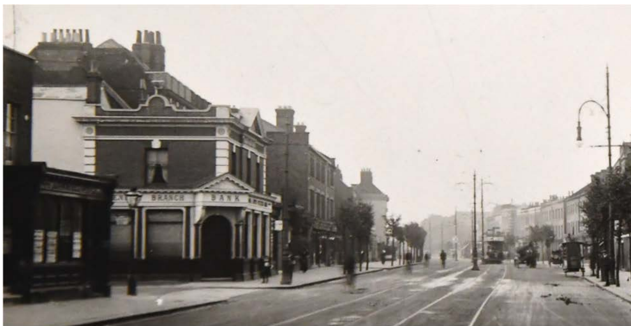
Figure 10 - Circa 1920 High Road looking from Number 814 towards the gable of 790 Dial House.
