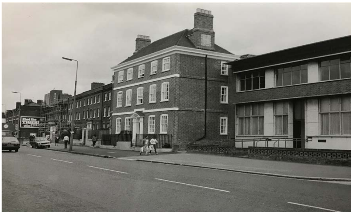
Figure 30 – After 1984 restoration of Dial House. Note the new window openings within the brick side elevation.
