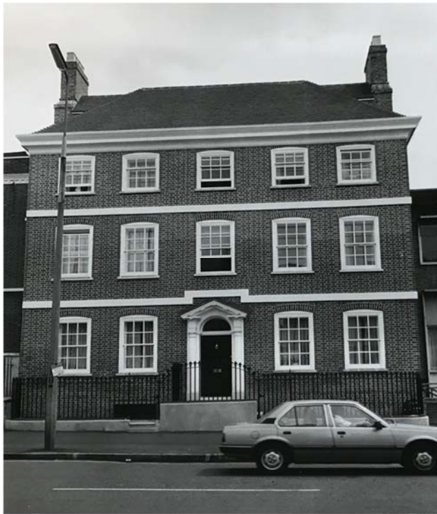
Figure 27 - July 1984 after restoration of Dial House with the roof and chimneys rebuilt and the windows reinstated to their Georgian proportions.
