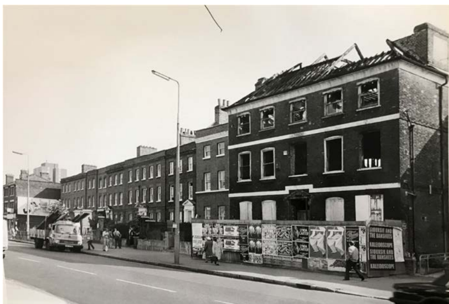
Figure 26 - Northumberland Terrace in September 1980 prior to repair of the fire damage.
