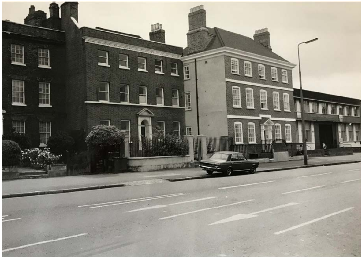
Figure 29 - Numbers 790 Dial House and 792 after restoration. Note the new window openings within the render side elevation of Dial House.
