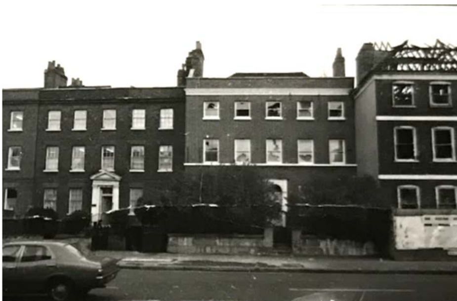
Figure 22 – Frontages of Numbers 790 to 794 in 1977 after the fire.
