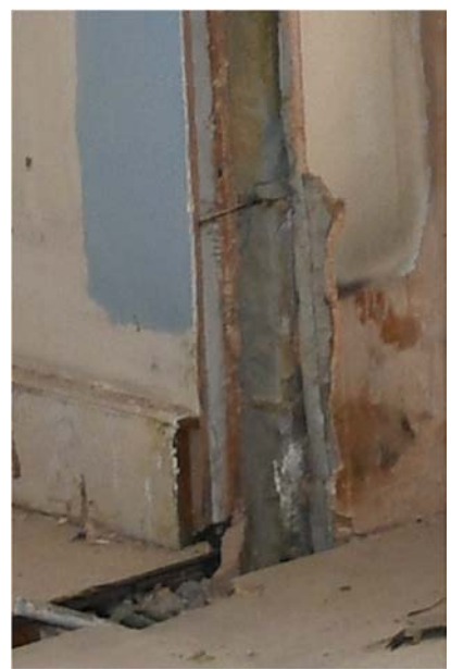
Figures 35a-b Above showing typical c1984 brick wall and plasterboard lining finish of the central Stair core. Photograph shows opening up on Ground Floor NW reception room South Wall.
