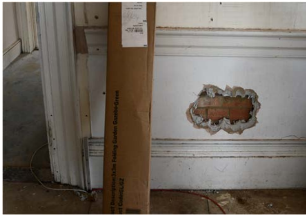
Figures 35a-b Above showing typical c1984 brick wall and plasterboard lining finish of the central Stair core. Photograph shows opening up on Ground Floor NW reception room South Wall.
