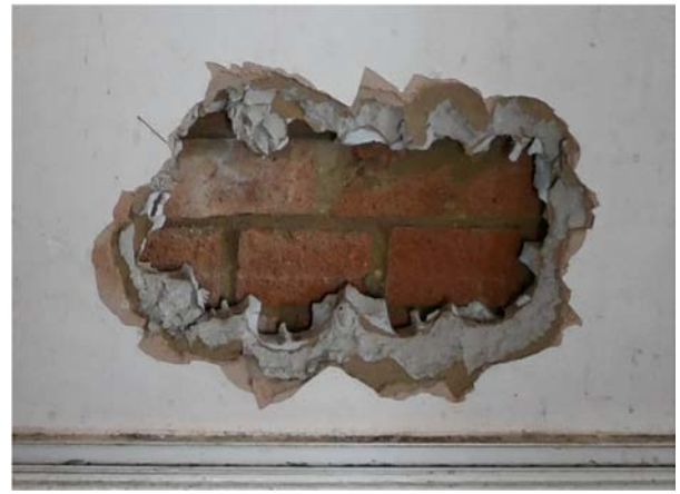
Figures 35a-b Above showing typical c1984 brick wall and plasterboard lining finish of the central Stair core. Photograph shows opening up on Ground Floor NW reception room South Wall.
