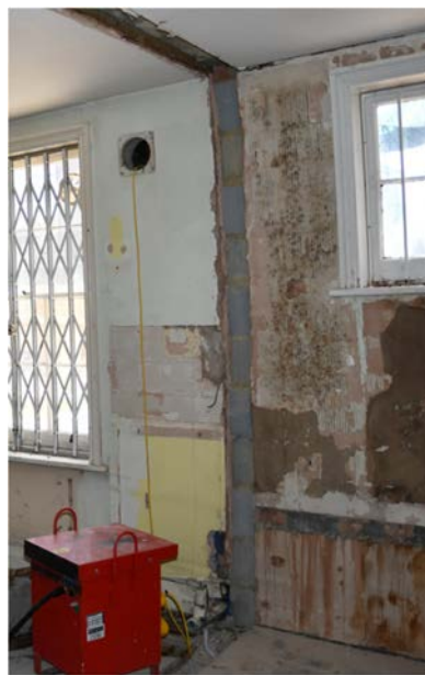
Figures 35a-b Above showing typical c1984 brick wall and plasterboard lining finish of the central Stair core. Photograph shows opening up on Ground Floor NW reception room South Wall.
