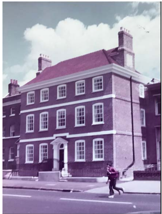
Figure 27 - July 1984 after restoration of Dial House with the roof and chimneys rebuilt and the windows reinstated to their Georgian proportions.
