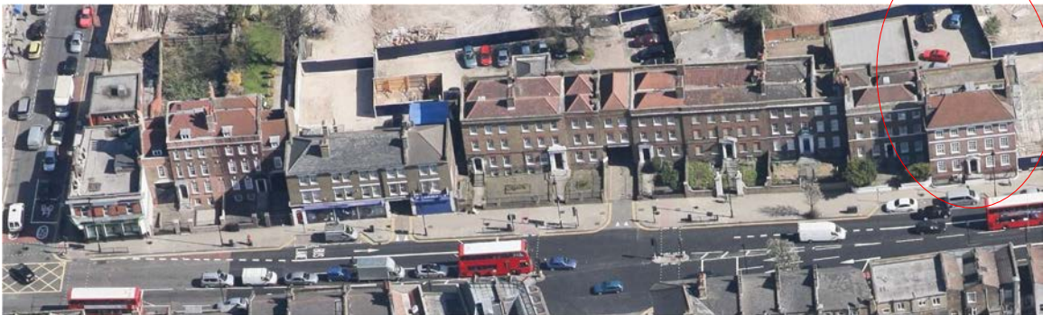
Figure 39 – 2013 Aerial of the Terrace prior to the construction of Lilywhite House.
