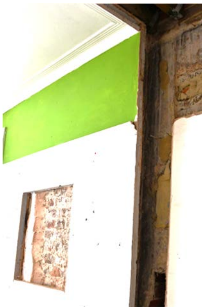
Figures 35a-b Above showing typical c1984 brick wall and plasterboard lining finish of the central Stair core. Photograph shows opening up on Ground Floor NW reception room South Wall.
