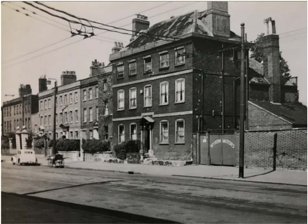
Figure 14 - 1952. Number 790 Dial House and Wyvern Motors in the foreground, showing the rear roof, chimney and lean-to.
